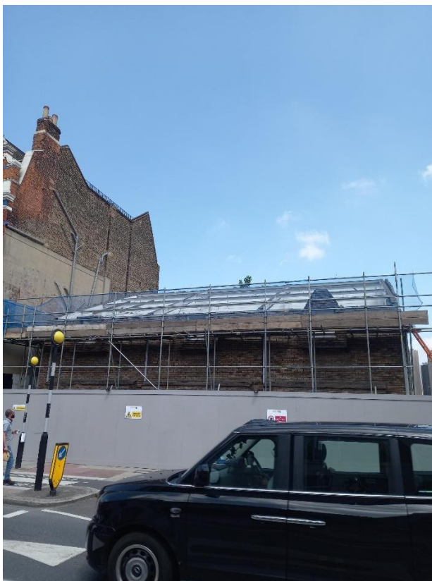
Roof Covering Removal
