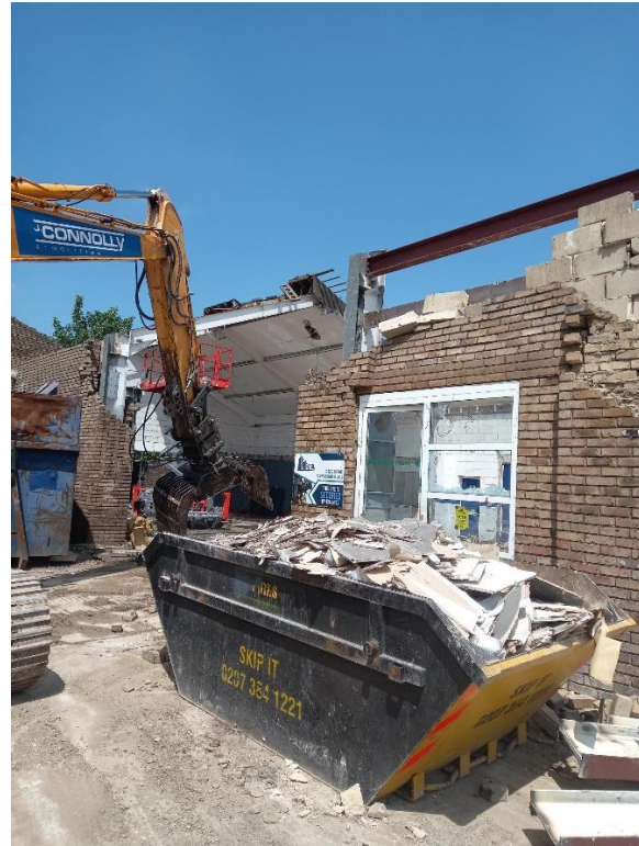
West Façade Demolition
