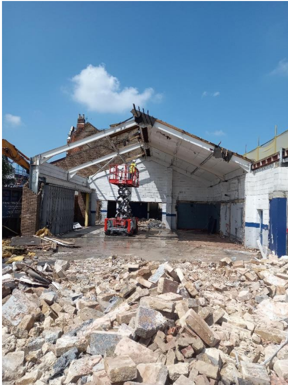
South Wall Demolition
