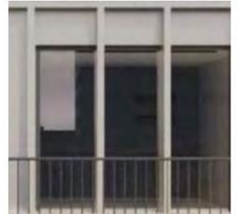
Wet-cast stone fins and spandrel to pavilion
