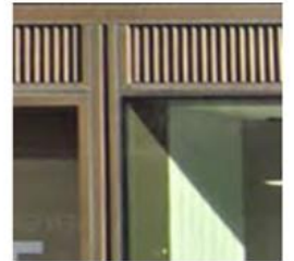
Metal grill and framed glazing
