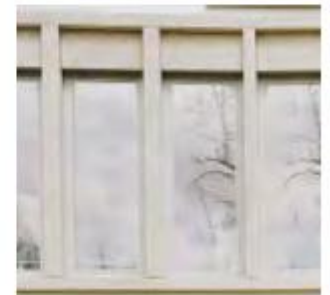
Stone surround to windows
