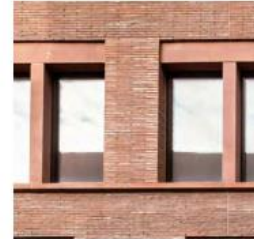
Wet-cast stone lintel to match brickwork
