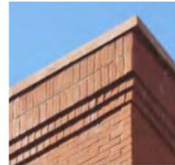
Soldier stack brick bonding at coping
