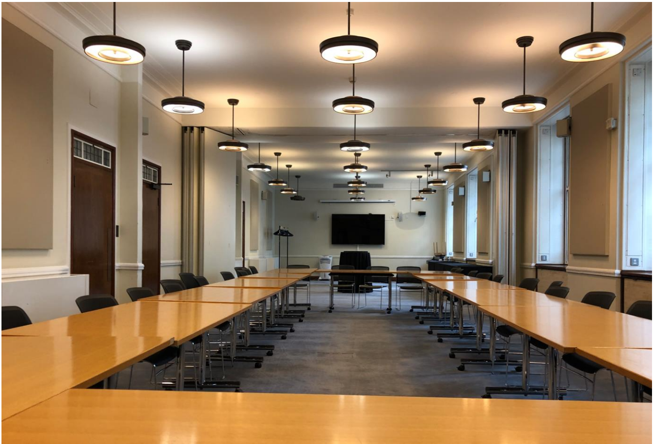
Photograph 2 – Existing acoustic panels fixed to external wall between windows.
