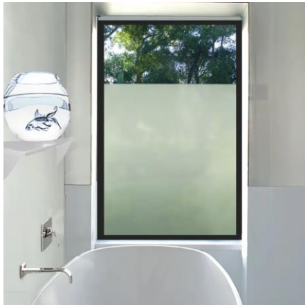
Photo showing example of obscure glazing
