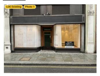
The existing entrance is formed of a wood frame housing a bay window arrangement and wood door. Whilst the wood is in reasonably good condition it offers no security protection having two standard 5 lever mortice locks and no disabled access facilities.
