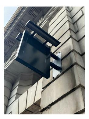
Existing plate and holes will be use not opening a new holes.
