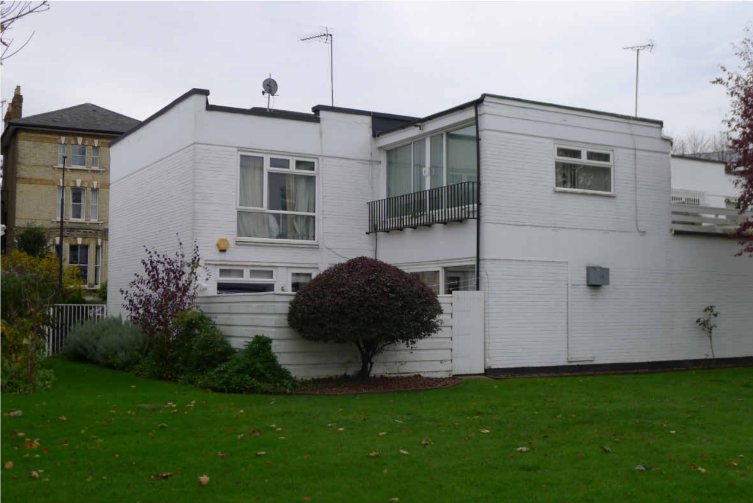
REAR ELEVATION FACING NORTH
