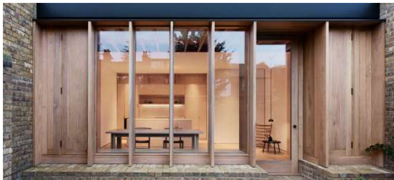
Deep timber framing to contemporary glazing
