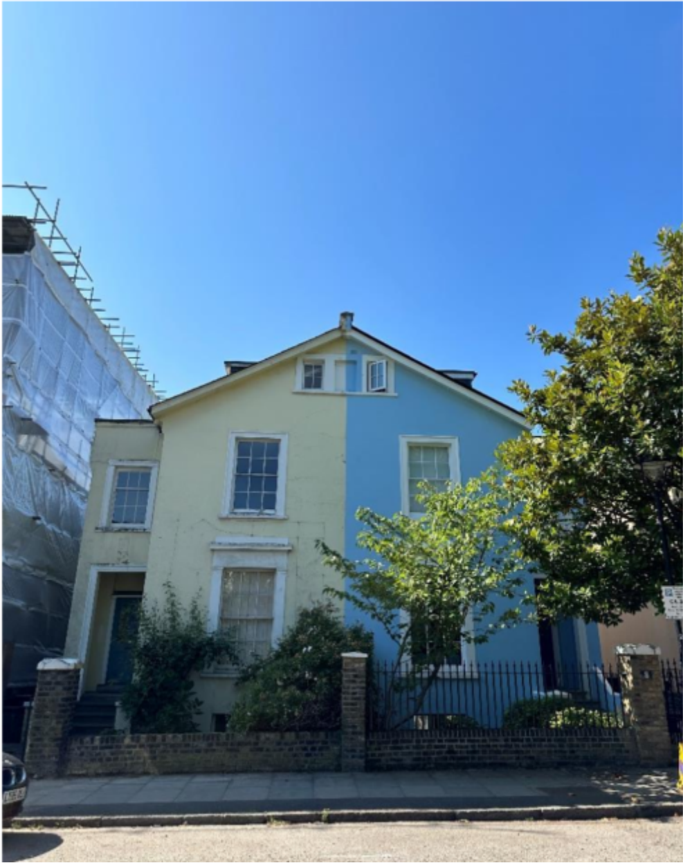
Image 2: streetview of front elevation. No 7 on the left.
