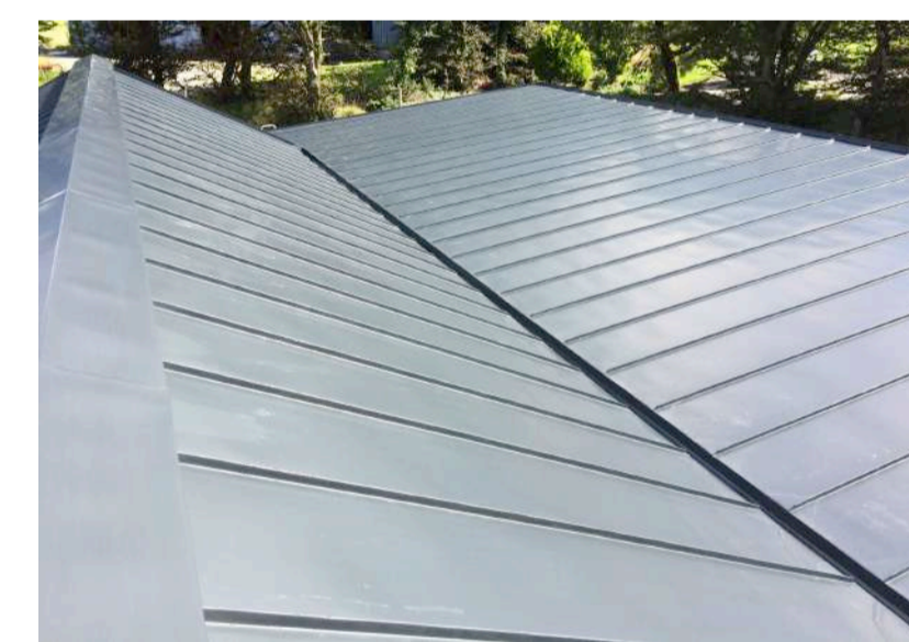
NATURAL ZINC STANDING SEAM ROOF MATERIALS NTS
