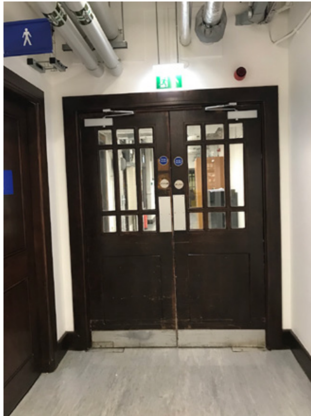
Photograph P3: Existing Door D.3.7
