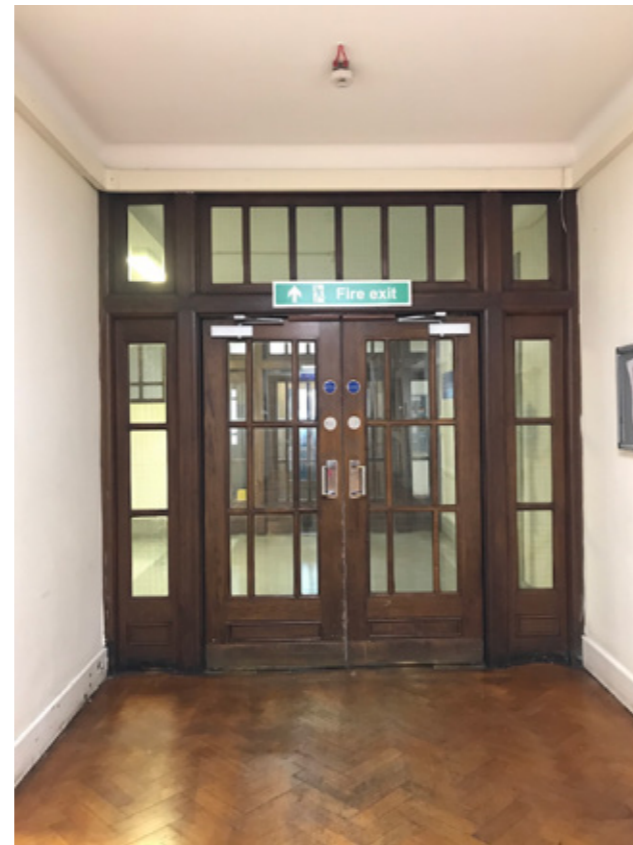
Photograph P2: Existing Door D.1.3 (Corridor Side)
