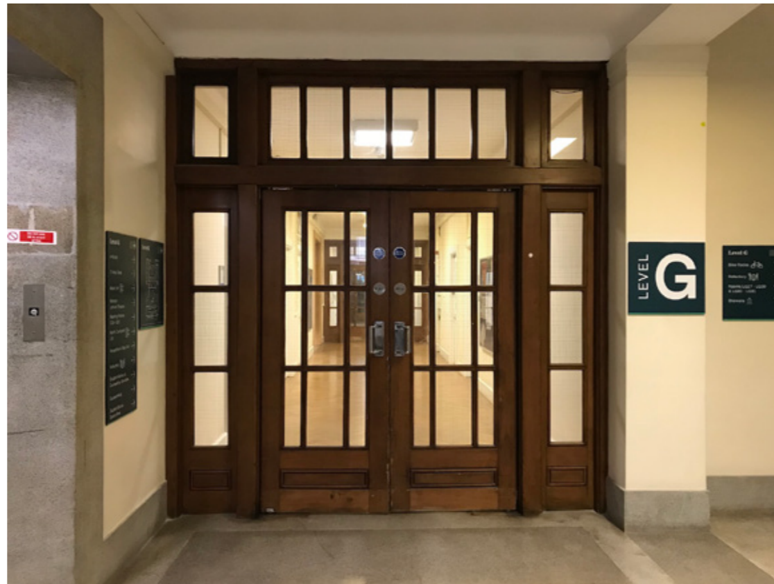
Photograph P1: Existing Door D.G.4 (Stair Core Side)
