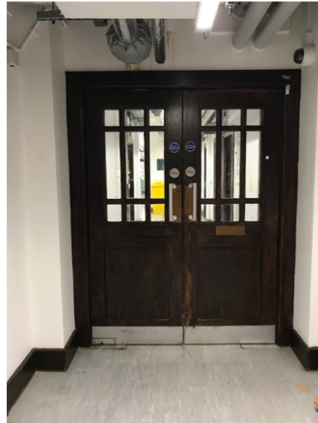
Photograph P4: Existing Door D.3.7
