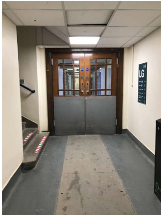
Photograph P1: Existing Door D.LG.3 (Stair Core Side)
