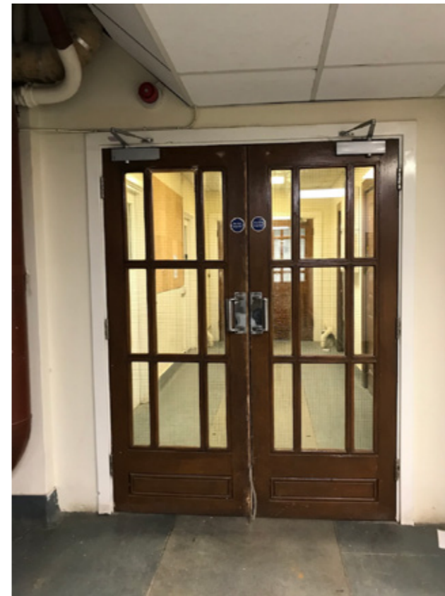
Photograph P3: Existing Door D.LG.4 (Stair Core Side)
