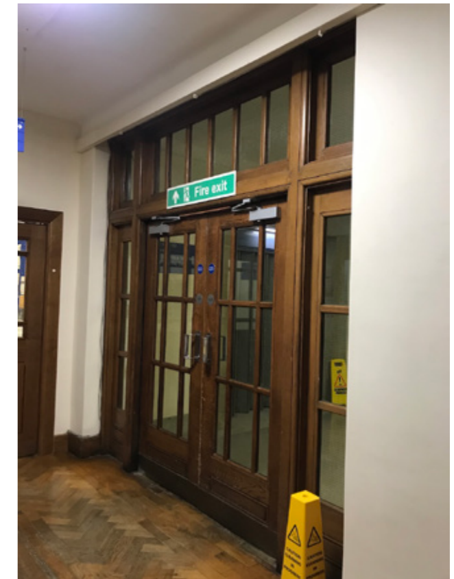
Photograph P4: Existing Door D.1.4 (Corridor Side)
