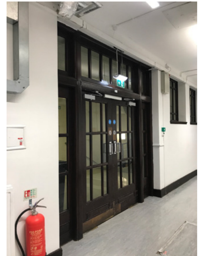
Photograph P4: Existing Door D.3.4 (Corridor Side)
