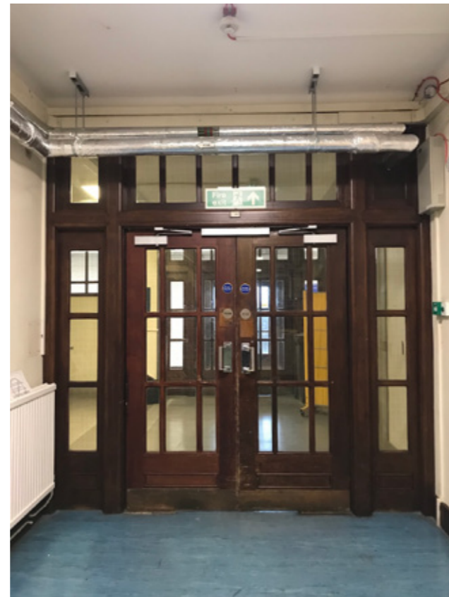
Photograph P2: Existing Door D.3.3 (Corridor Side)
