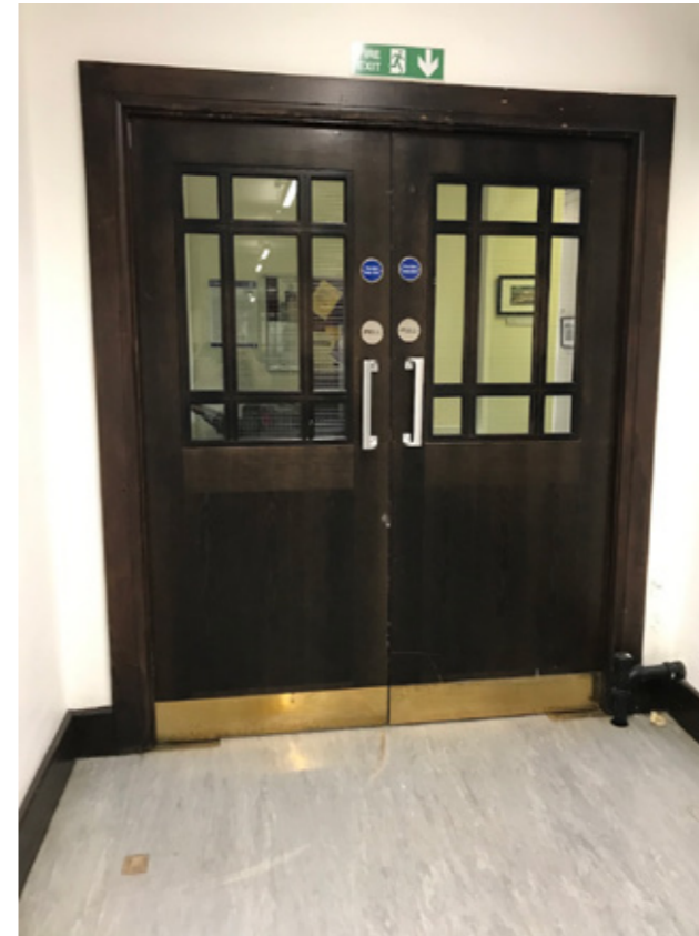
Photograph P5: Existing Door D.3.8
