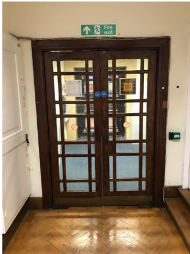
Photograph P3: Existing Door D.17 (Corridor Side)
