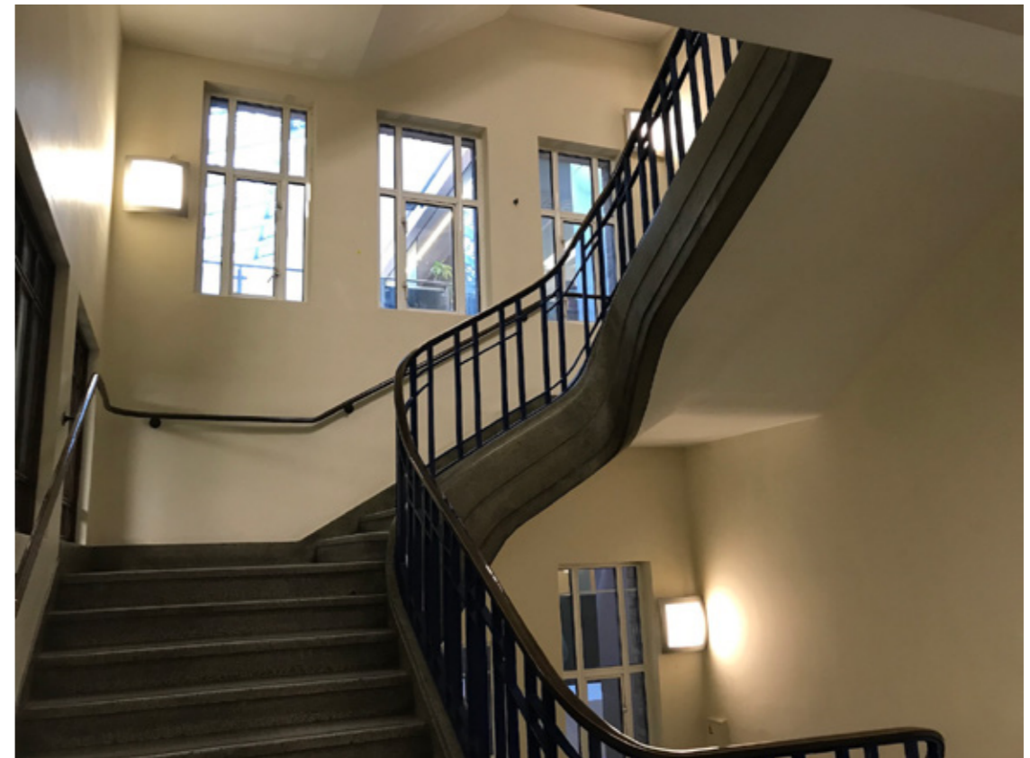
Photograph P5: Stair Core 2 South-East Elevation: Existing Windows Above Third Floor
