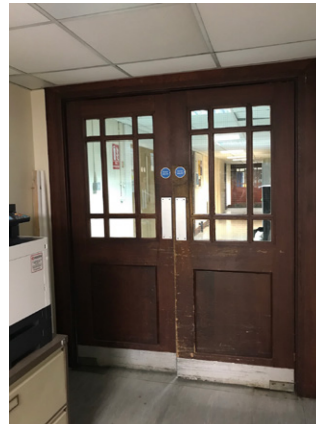
Photograph P1: Existing Door D.2.3
