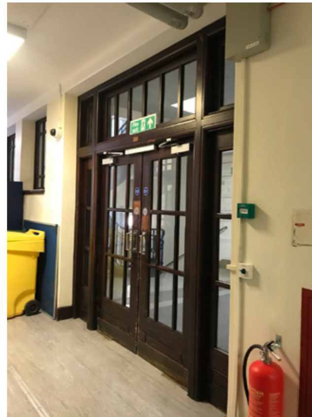
Photograph P2 Existing Door D.3.1 (Corridor Side)
