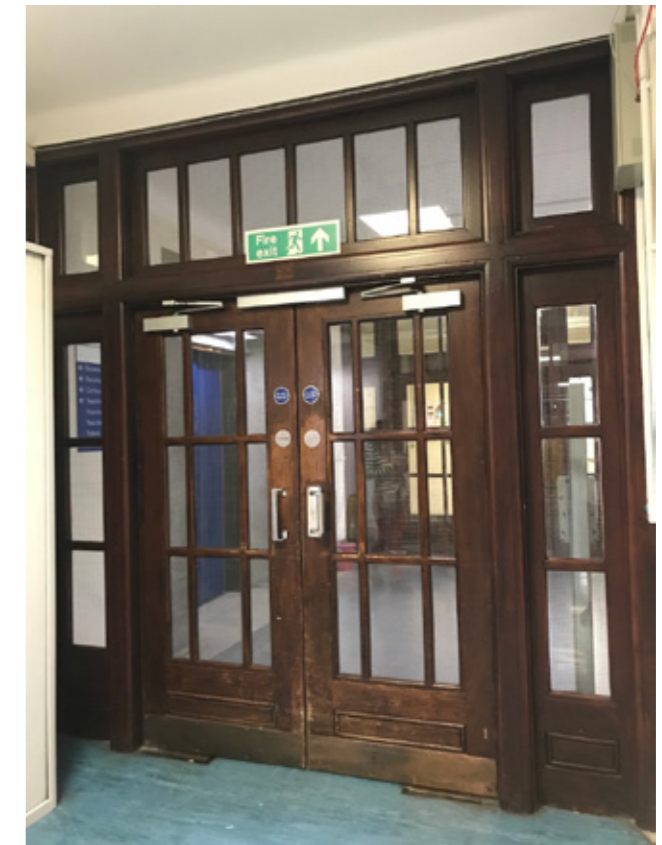
Photograph P4: Existing Door D.3.2 (Corridor Side)
