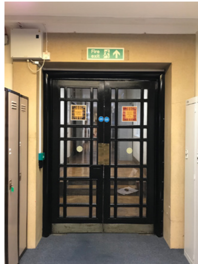
Photograph P4: Existing Door D.17 (Library Lobby Side)
