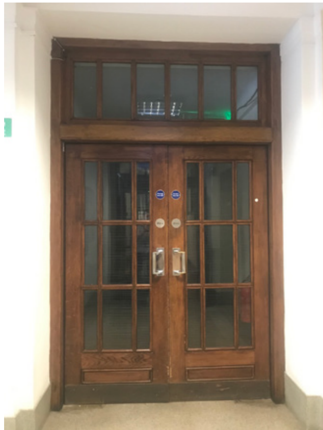
Photograph P3: Existing Door D.G.5 (Stair Core Side)
