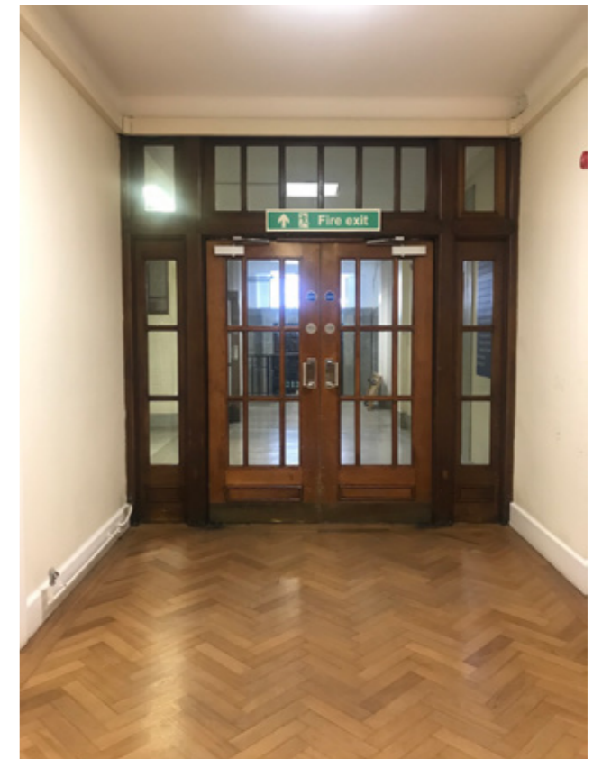
Photograph P2: Existing Door D.G.4 (Corridor Side)
