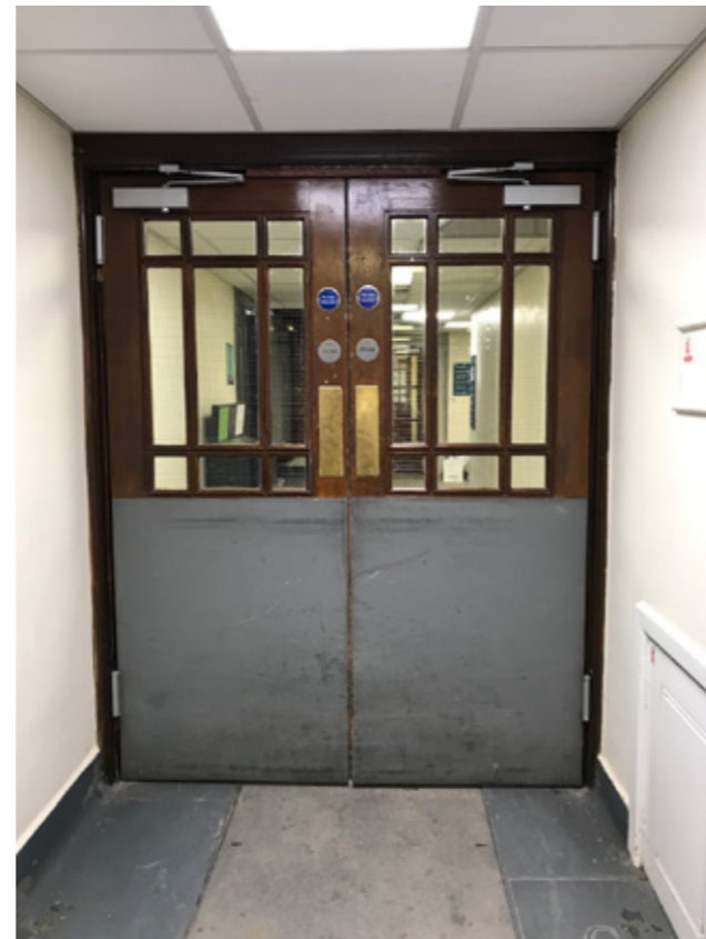
Photograph P2 Existing Door D.LG.3 (Corridor Side)
