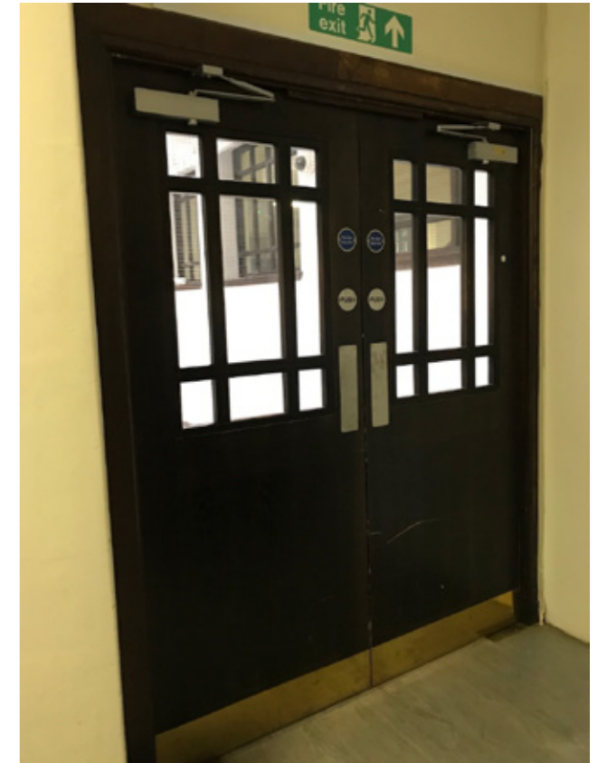
Photograph P6: Existing Door D.3.8
