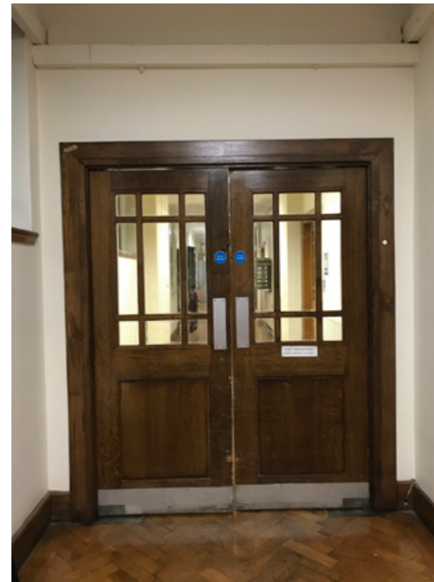
Photograph P1: Existing Door D.16
