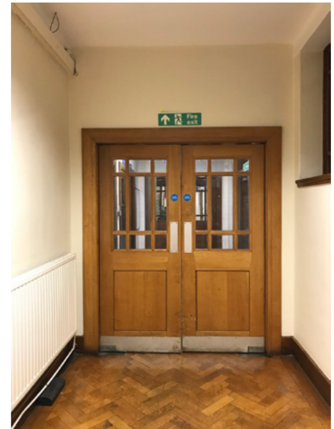
Photograph P2: Existing Door D.16
