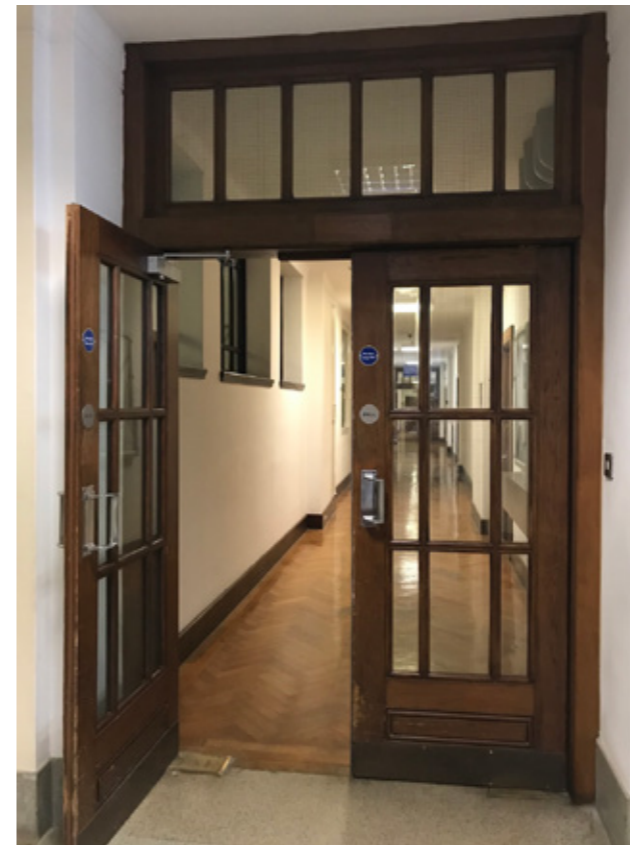
Photograph P5: Existing Door D.G.6 (Stair Core Side)
