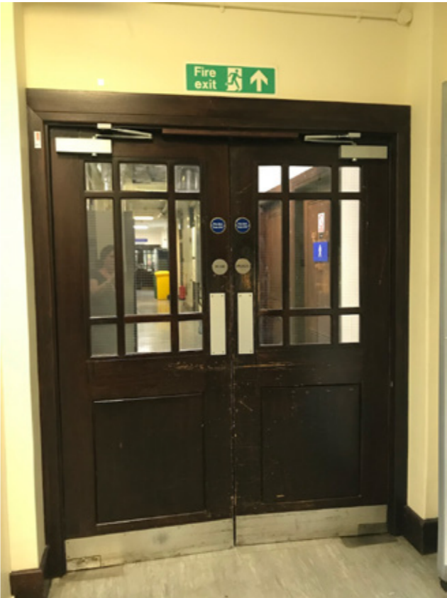
Photograph P1: Existing Door D.3.6
