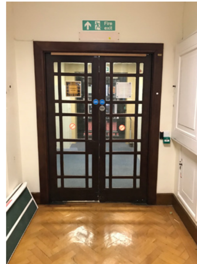
Photograph P5: Existing Door D.18 (Corridor Side)
