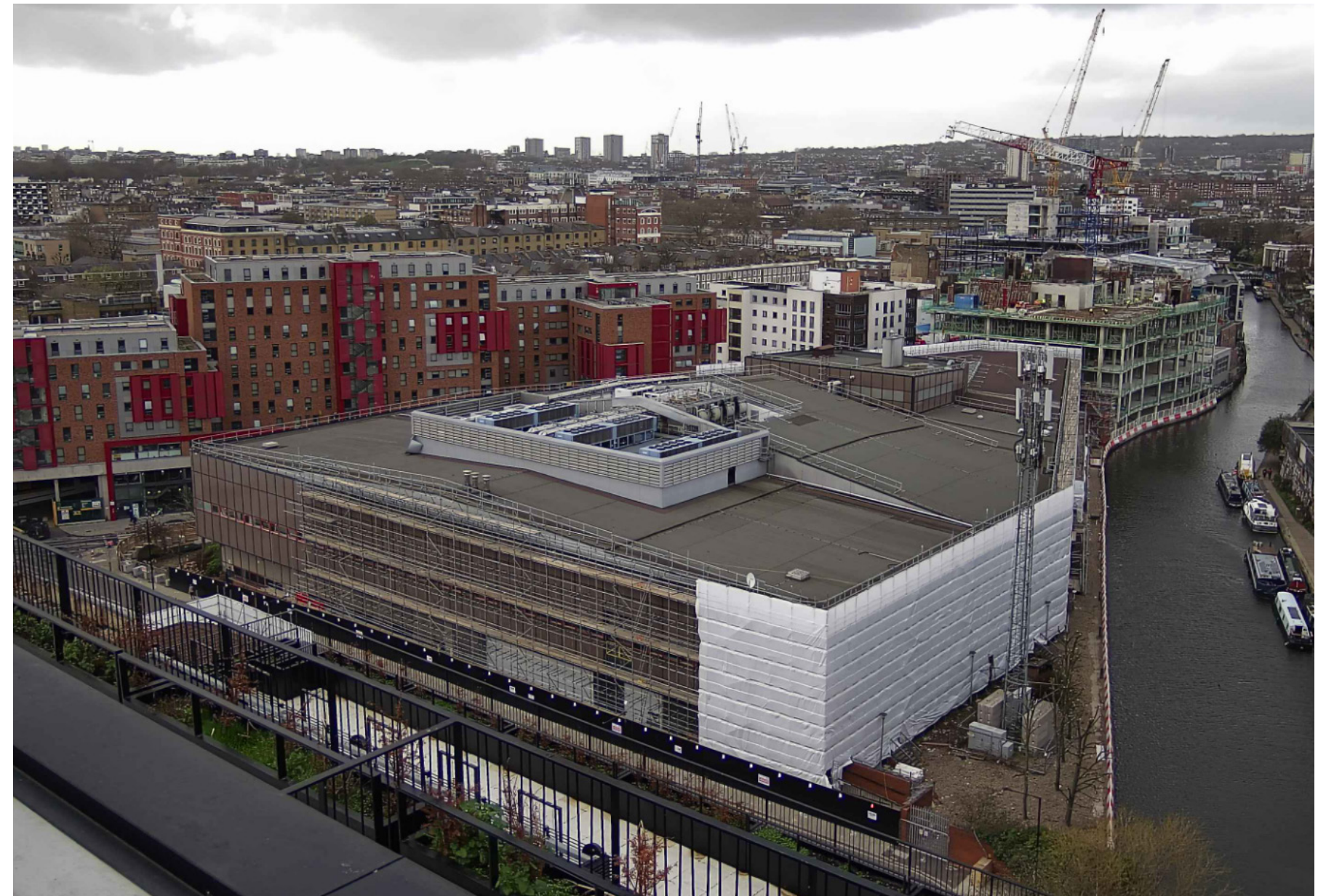
Ugly Brown Building, Pre Demolition, March 2023
