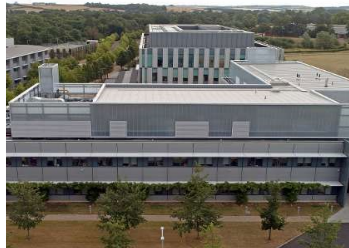
Example Building: Roof Following Conversion to Laboratory Use with Significant Expansion of Roof Plant Space
