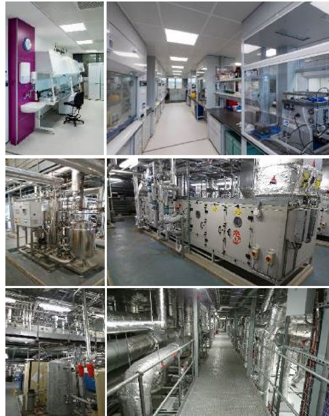
Typical Laboratory and Plant Equipment / Areas
