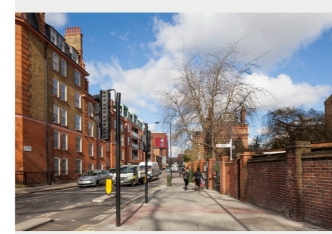
12 | St Pancras Way, junction with Pancras Road
