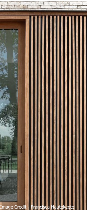
Timber Cladding
