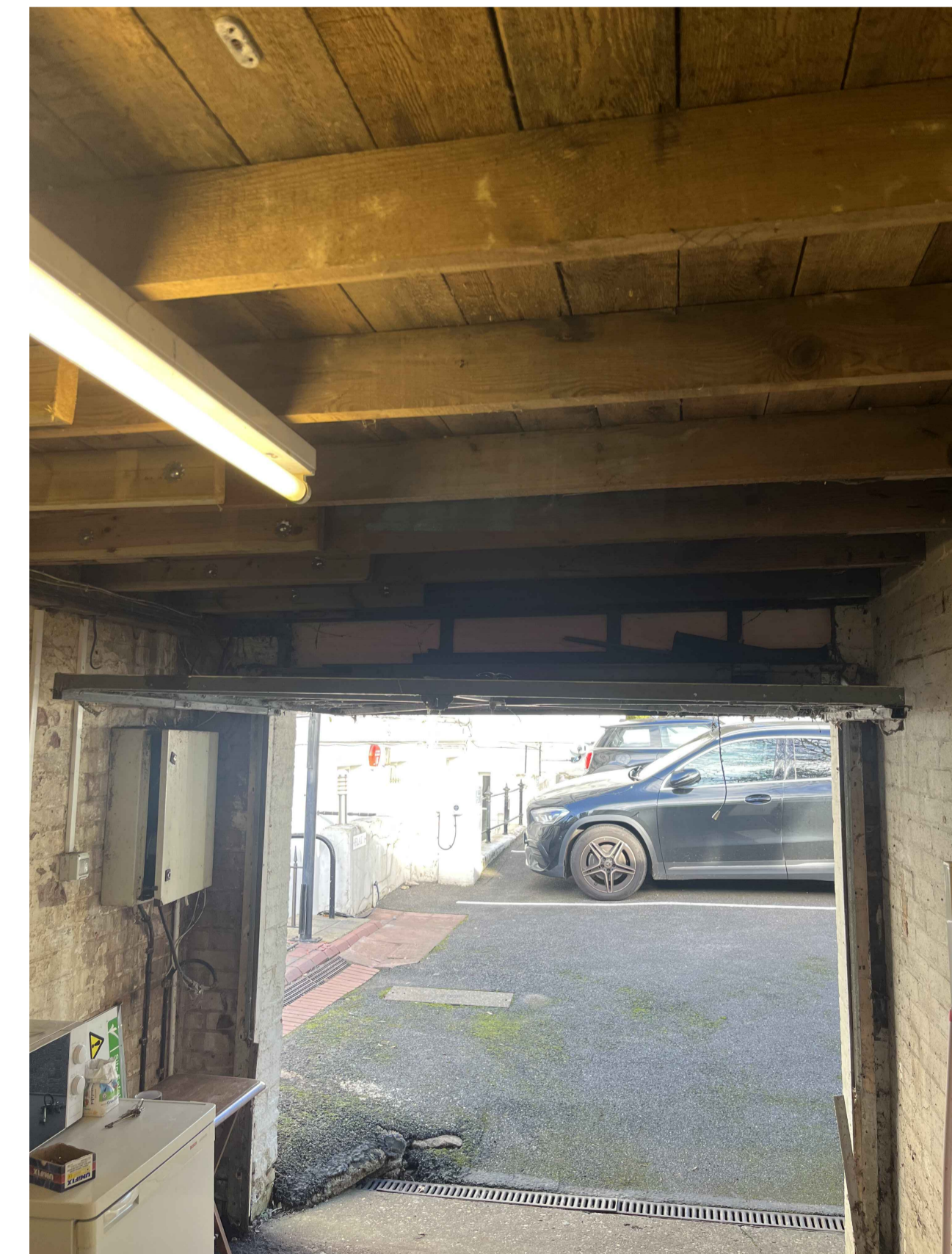
Image 6 : Typical void above garage doors
