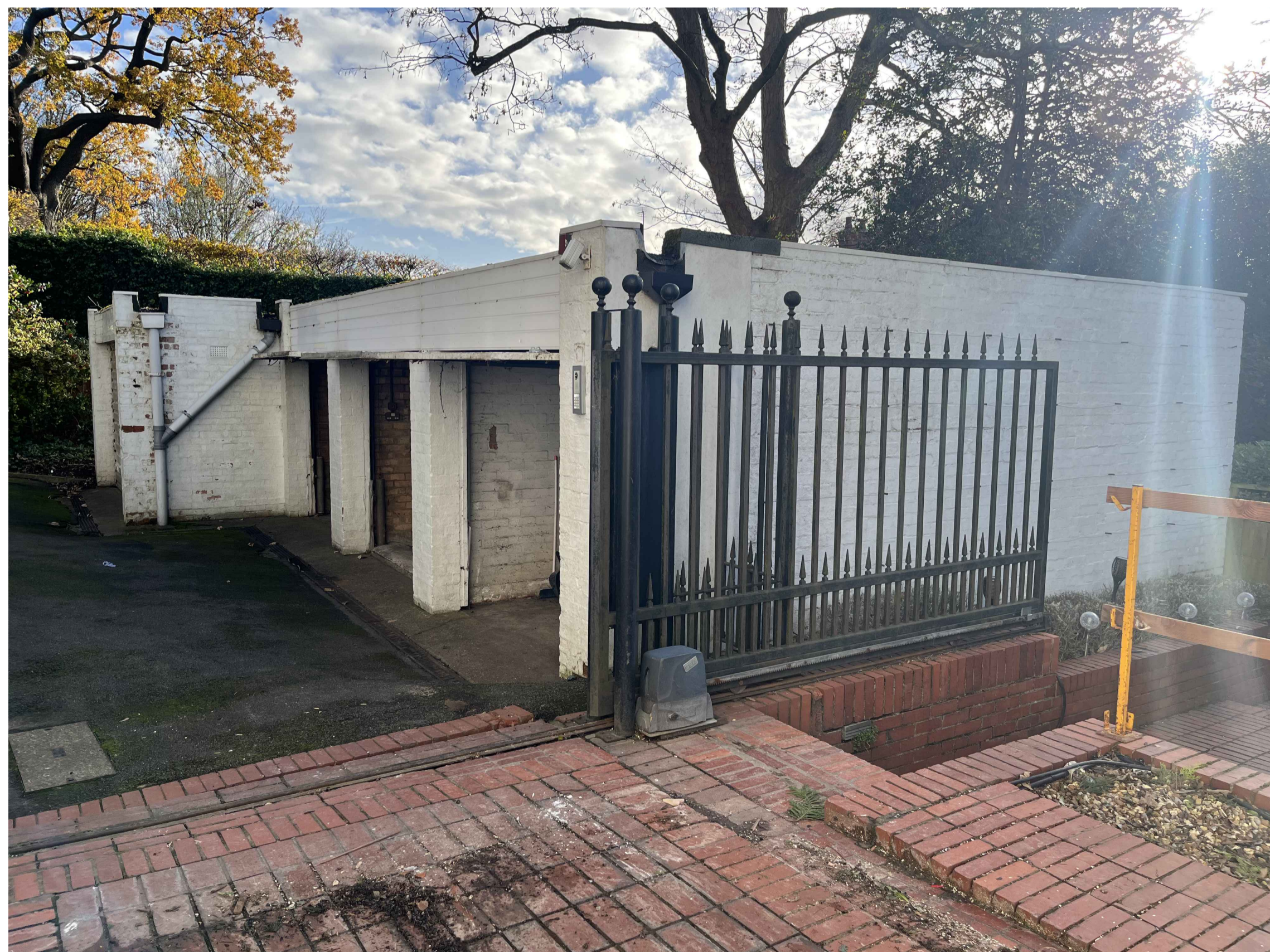
Image 4 : External view of stand-alone garages with doors open
