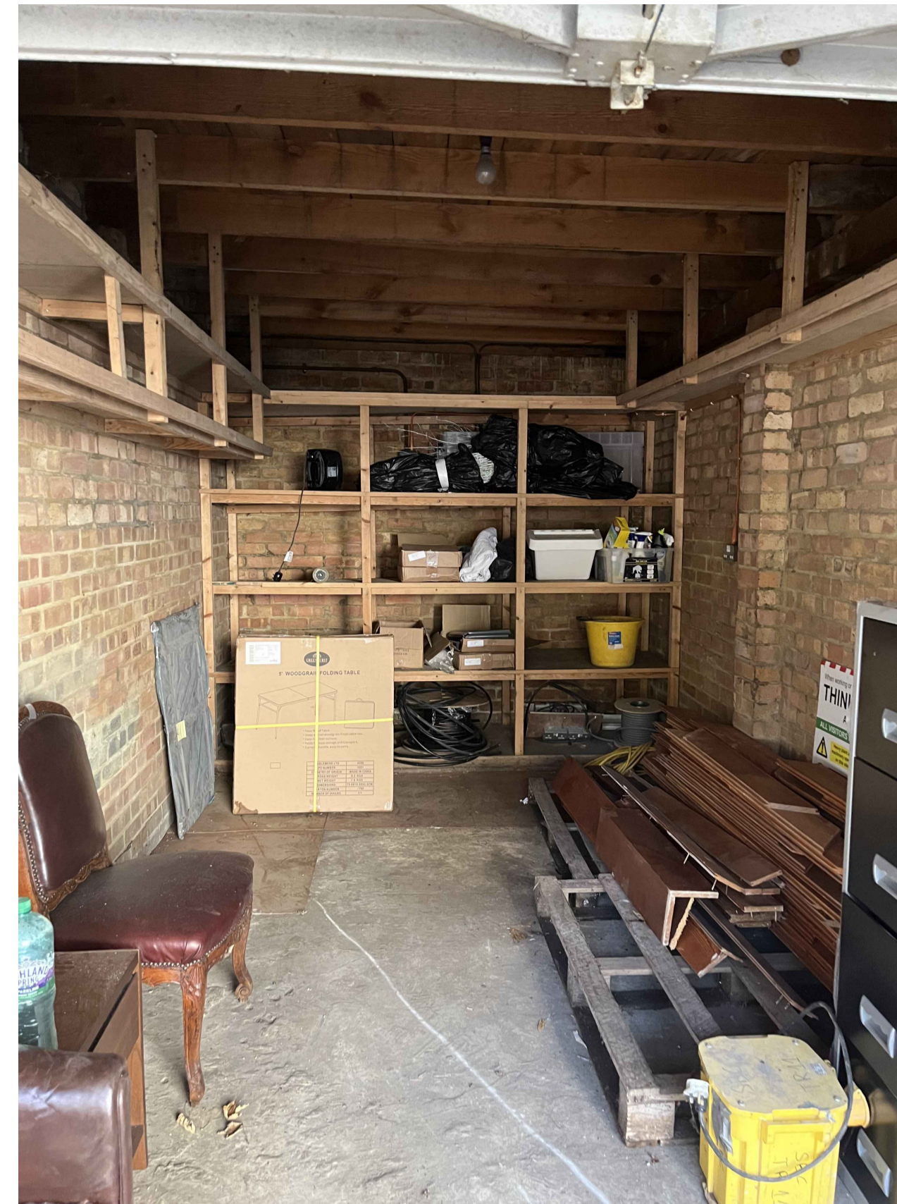
Image 2 : Internal view of garage 2
