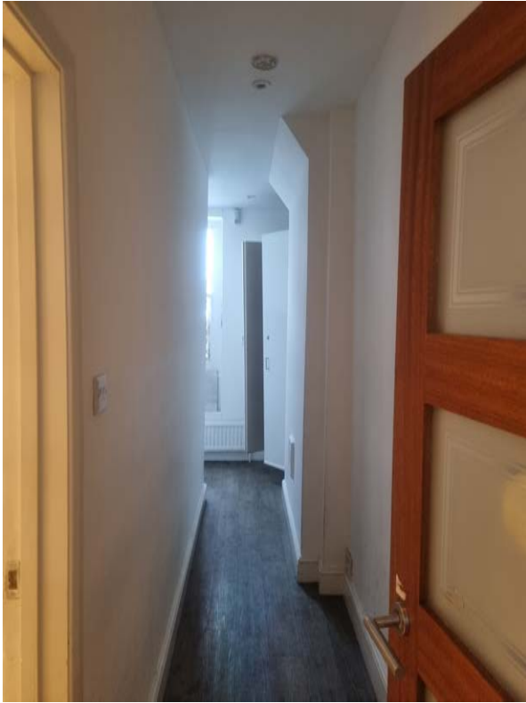
Ground floor level corridor looking towards the rear. The corridor is too narrow to form part of a fire escape route.
