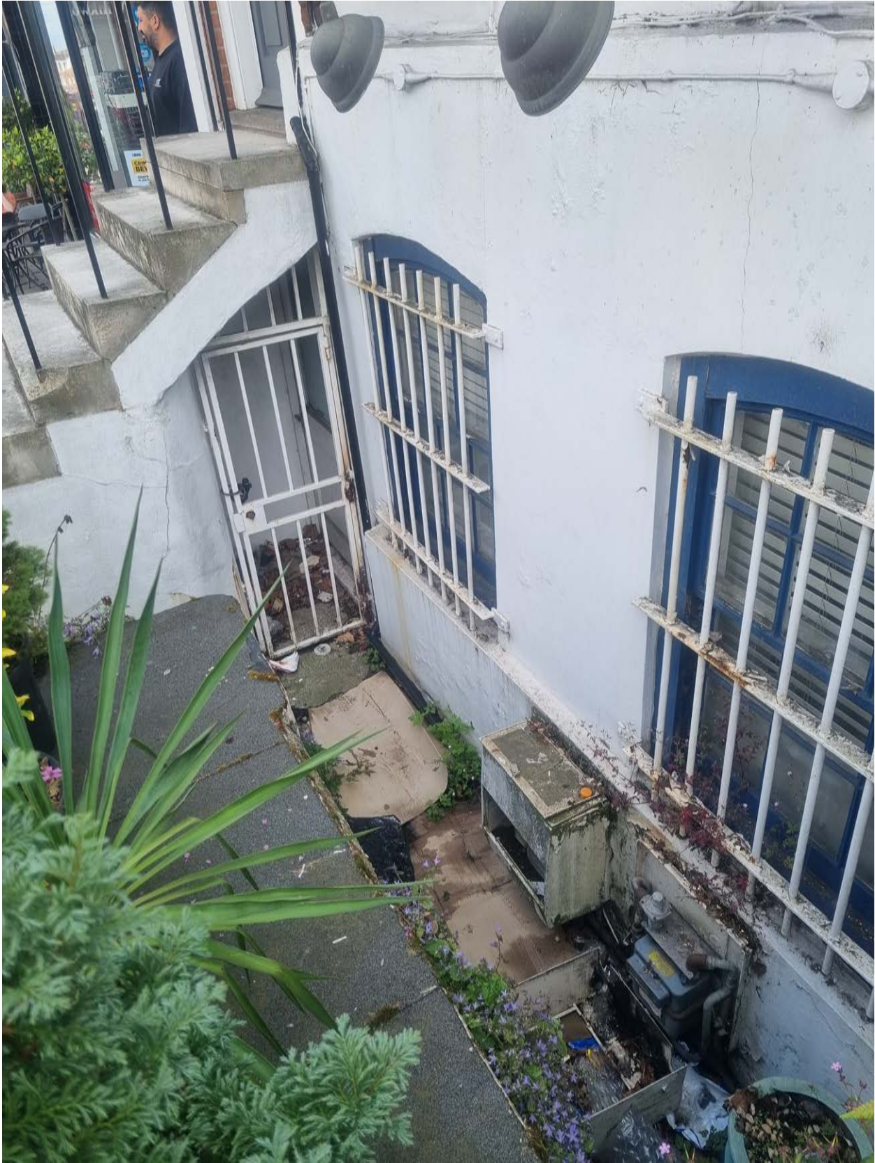
Entrance to 17b. The entrance is located below the stairs. Headroom is less than 2m under the stairs and at the threshold.
