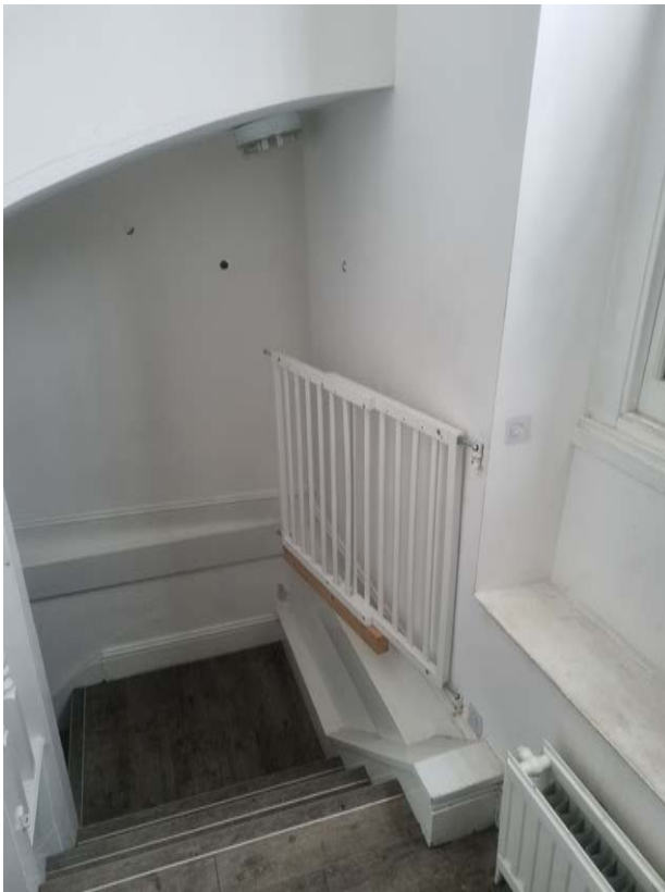
Ground floor – top of stairs. The headroom over the stairs is less than 2m.
