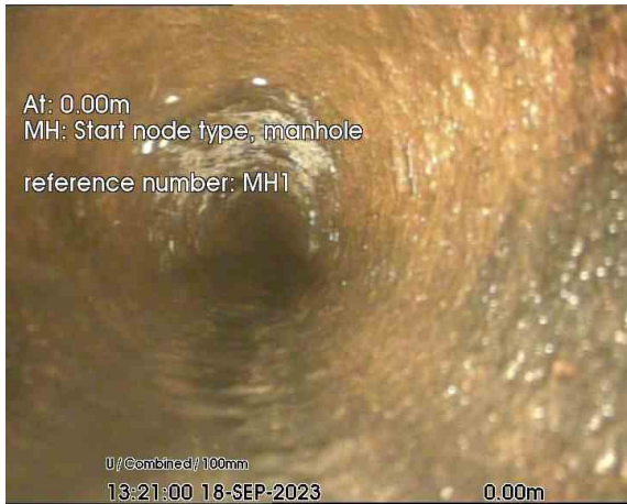
4_0-00m_132100.jpg, 00:00:00, 0.00 m Start node, manhole, reference: MH1
