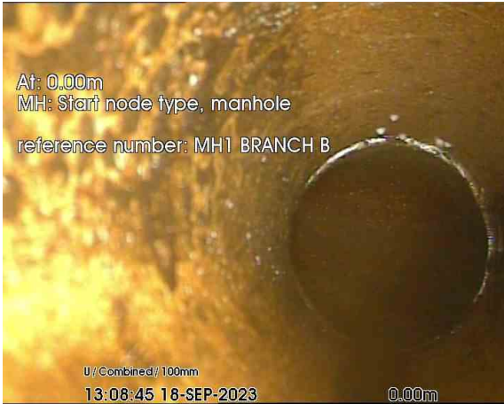
2_0-00m_130845.jpg, 00:00:00, 0.00 m Start node, manhole, reference: MH1 BRANCH B
