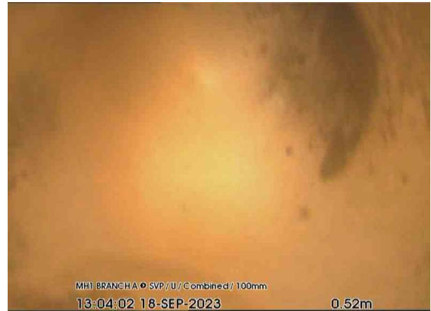
SVPX_fe5b9e2a-778d-49eb-99d7-b7ec33b6d1b9_20230921_150125_099.jpg, 00:00:23, 0.52 m Line deviates up
