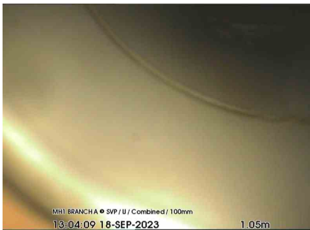
SVPX_d22d88ea-ddc7-43ae-ba32-71806bb7859f_20230921_150142_131.jpg, 00:00:31, 1.05 m Pipe material changes to polyvinyl chloride at this point
