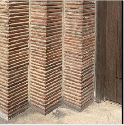
Brick tile reveal example
