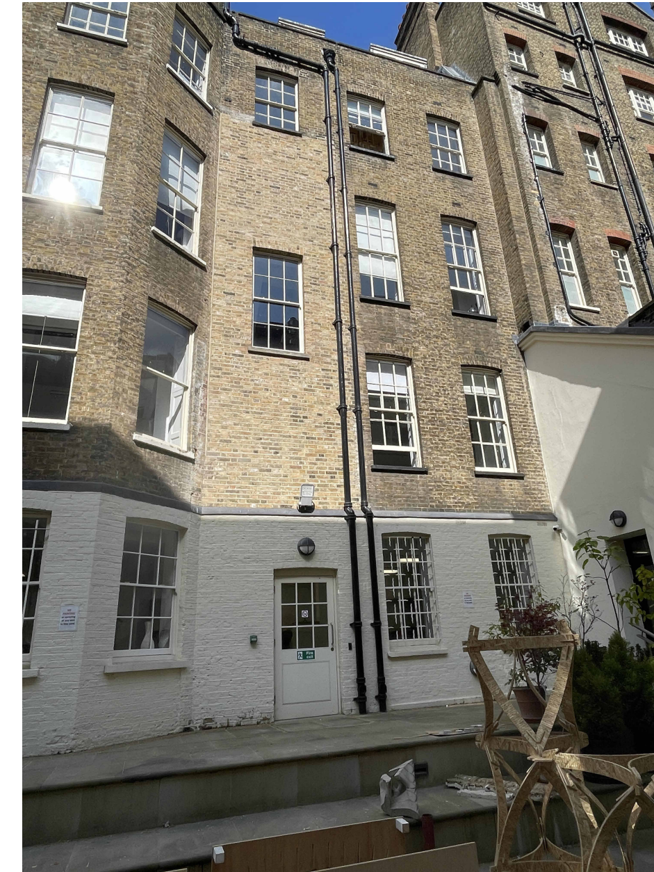
Existing Rear Elevation photo
