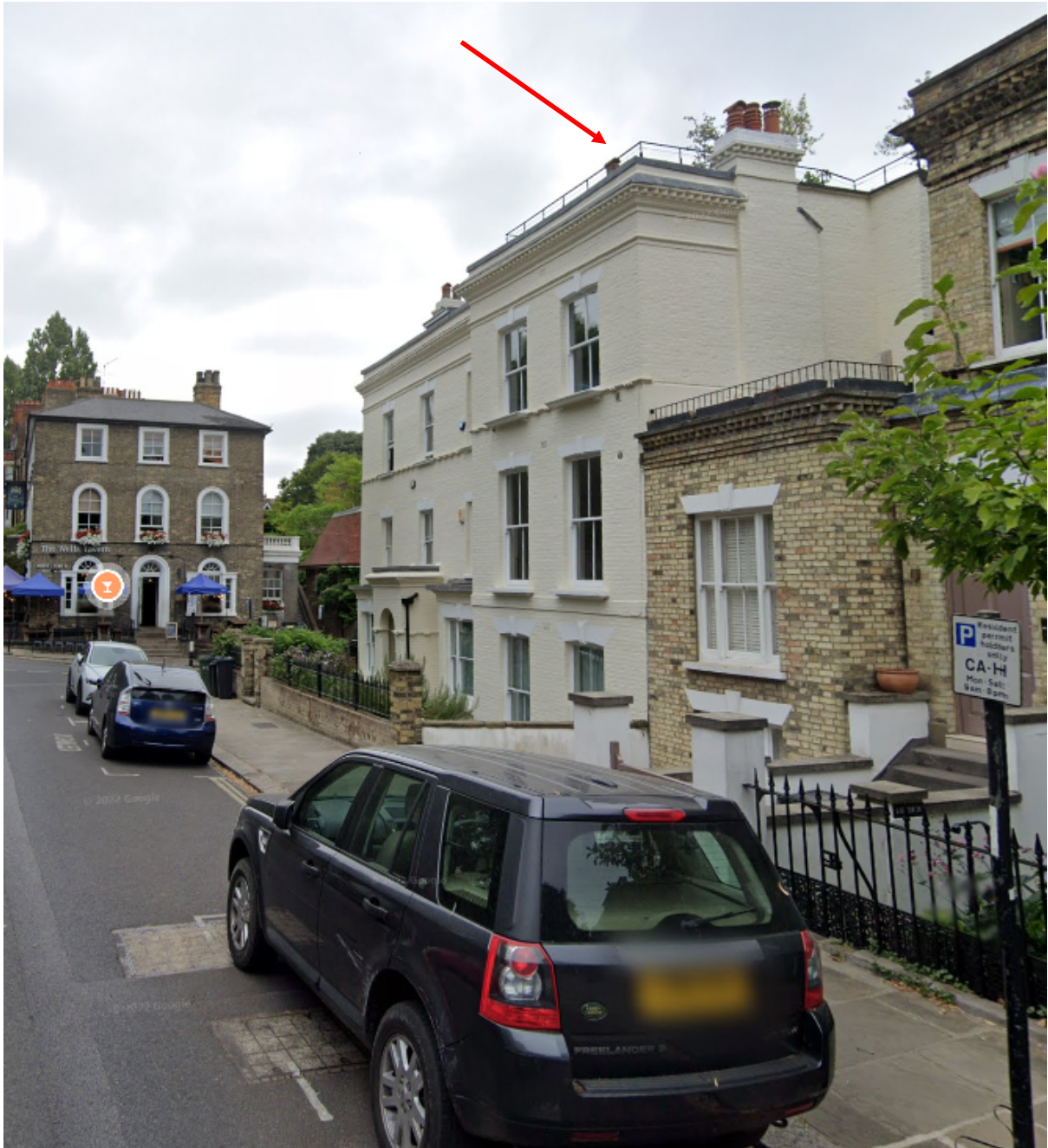
Photo 3: view looking north down Well Walk. Red arrow denotes area of roof extension
