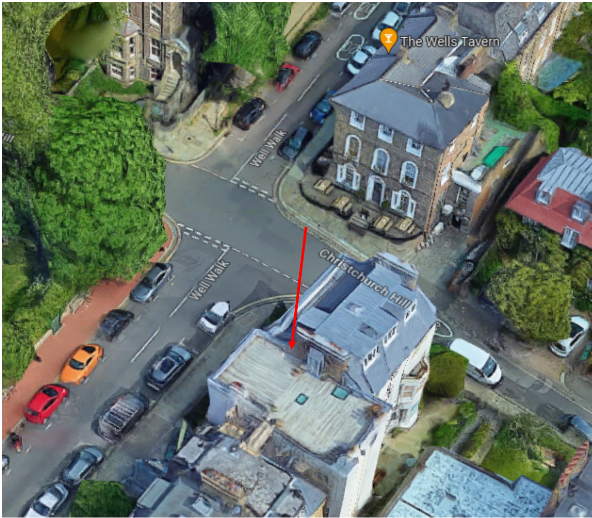
Photo 1: Aerial view of site. Red line denotes flat roof to be extended
