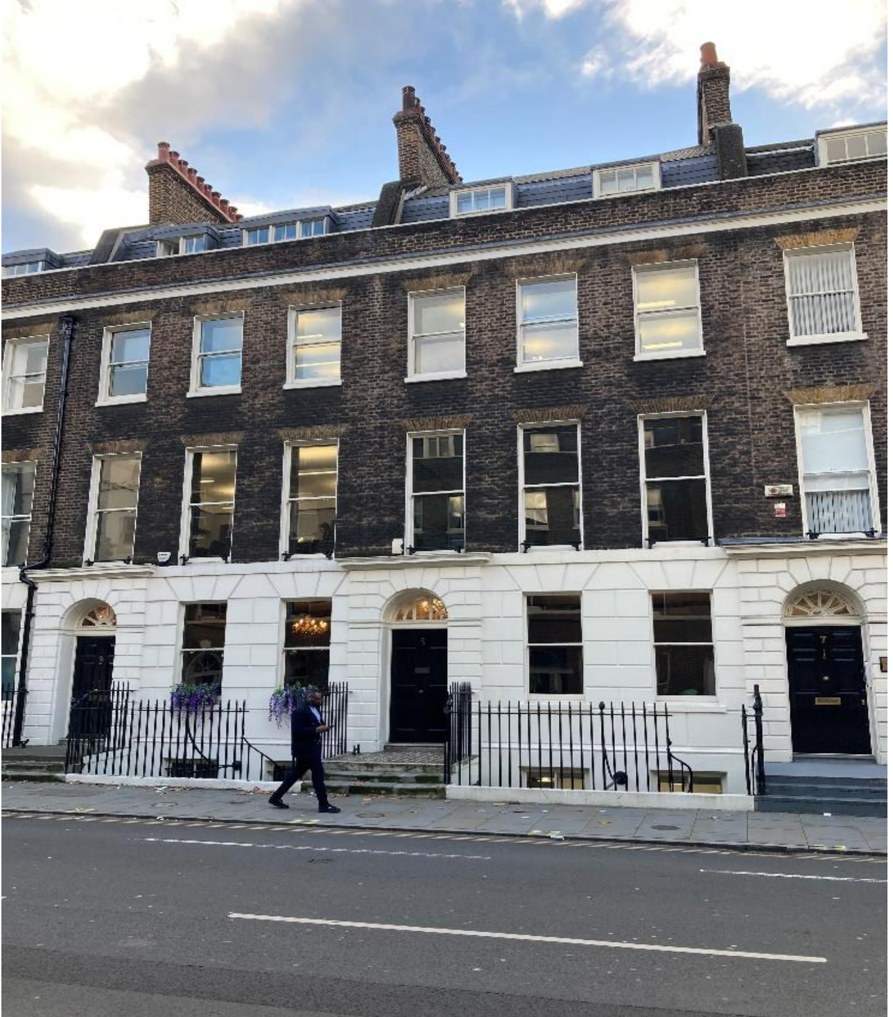
Figure 3.2 – Exterior of 3 and 5 Gower Street.
