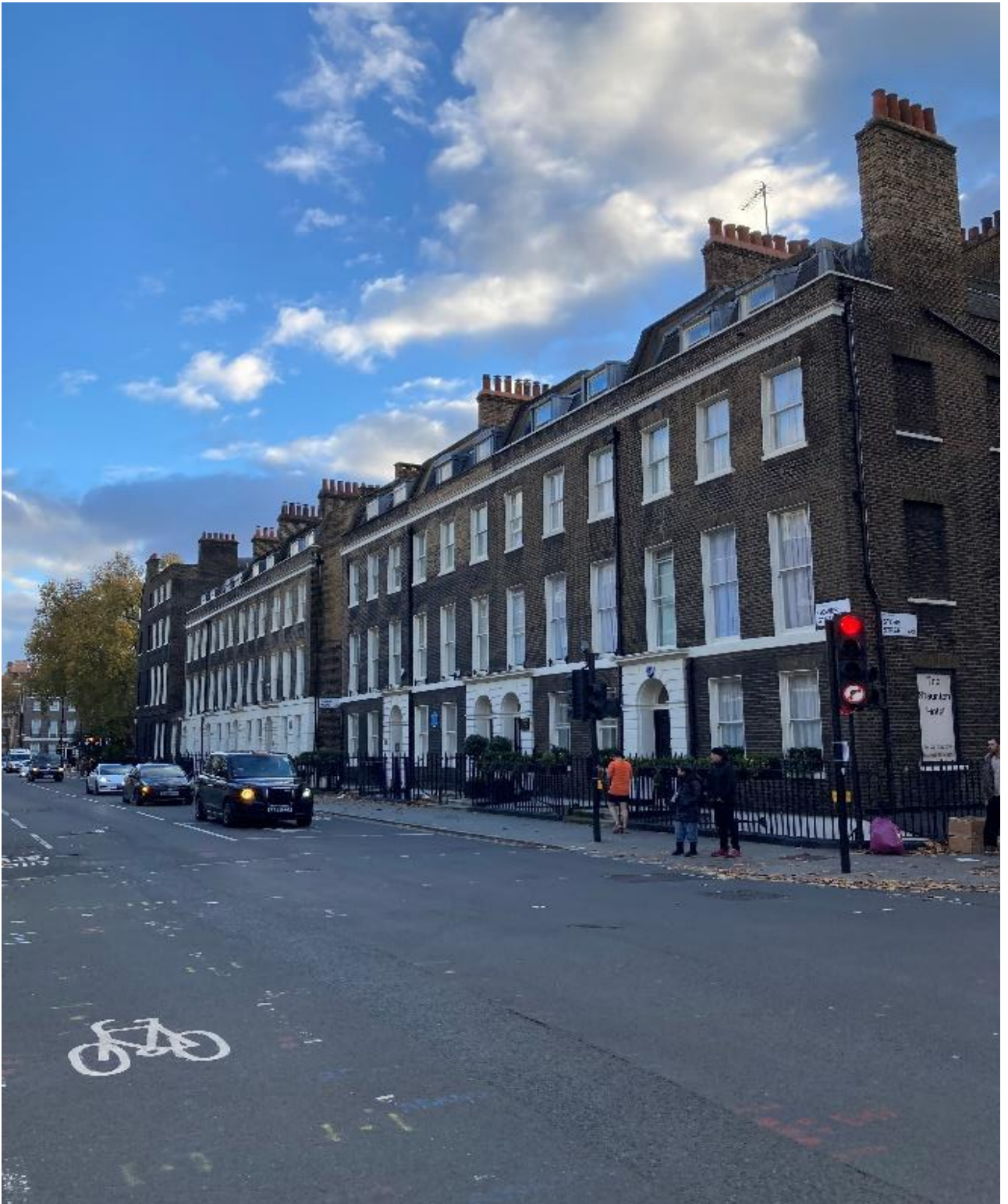
Figure 3.1 – View of the terrace at 1-15 Gower Street.
