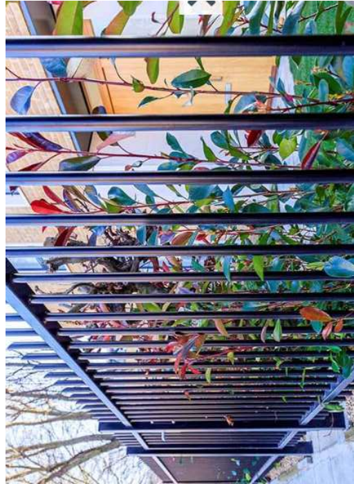
Steel vertical bar fence and gates PPC finish RAL 9005 (black)
