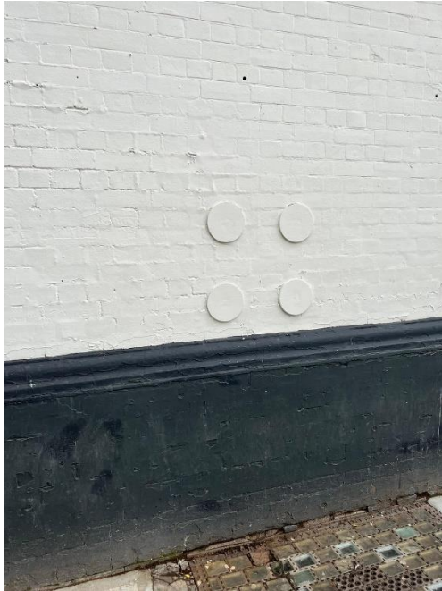
Figure 5-3 - Photograph of generator terminal element
