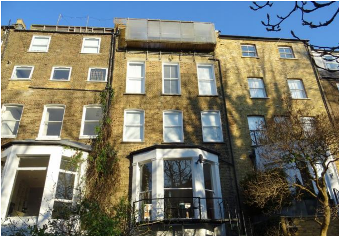
Photos 3 (above): Existing rear elevation
