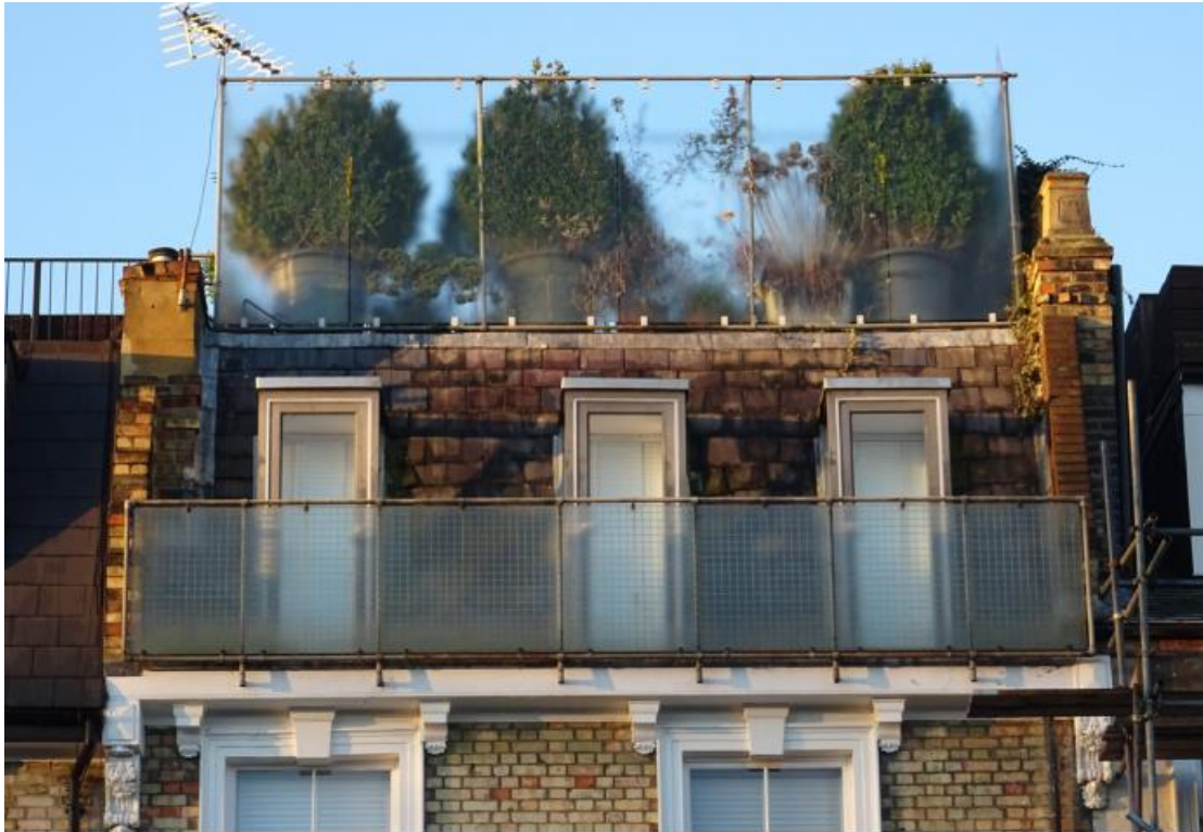
Photo 2 (above): Existing front elevation 3 rd floor balustrade and roof terrace balustrade
