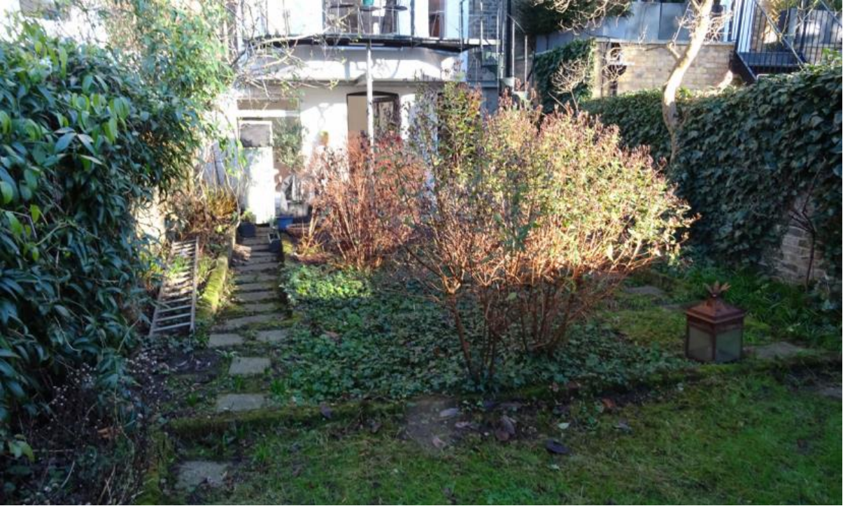
Photo 4 (above): Existing rear elevation showing lower ground floor
