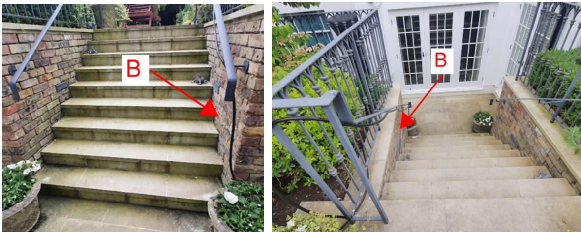
Images 10 & 11 – showing proposed stair lift location at rear of site (B) (looking up and down the rear stairs respectively)
