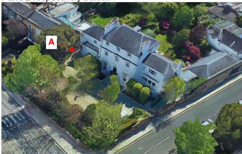
Image 1 – showing proposed stair lift location (A) at front (south side) of application site
