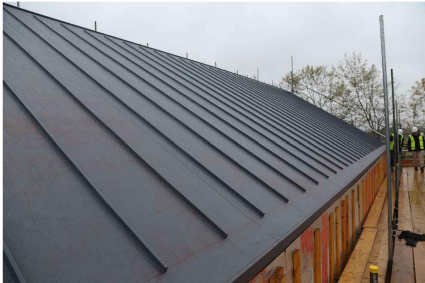
ILLUSTRATIVE EXAMPLE OF SINGLE PLY MEMBRANE ROOF WITH STANDING SEAM DETAIL, TO BE SPACED TO REPLICATE EXISTING ROOF PROFILE
