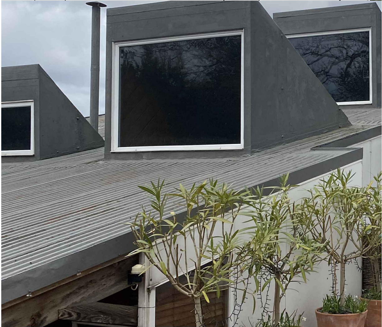
EXISTING RIBBED METAL ROOF IN POOR STATE OF REPAIR
