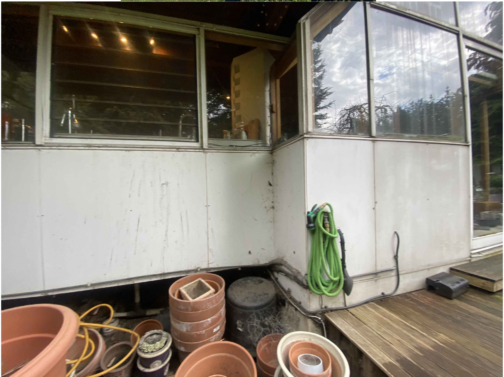
EXISTING FAILING WHITE COMPOSITE ALUMINIUM CLAD SINGLE GLAZED TIMBER WINDOWS
