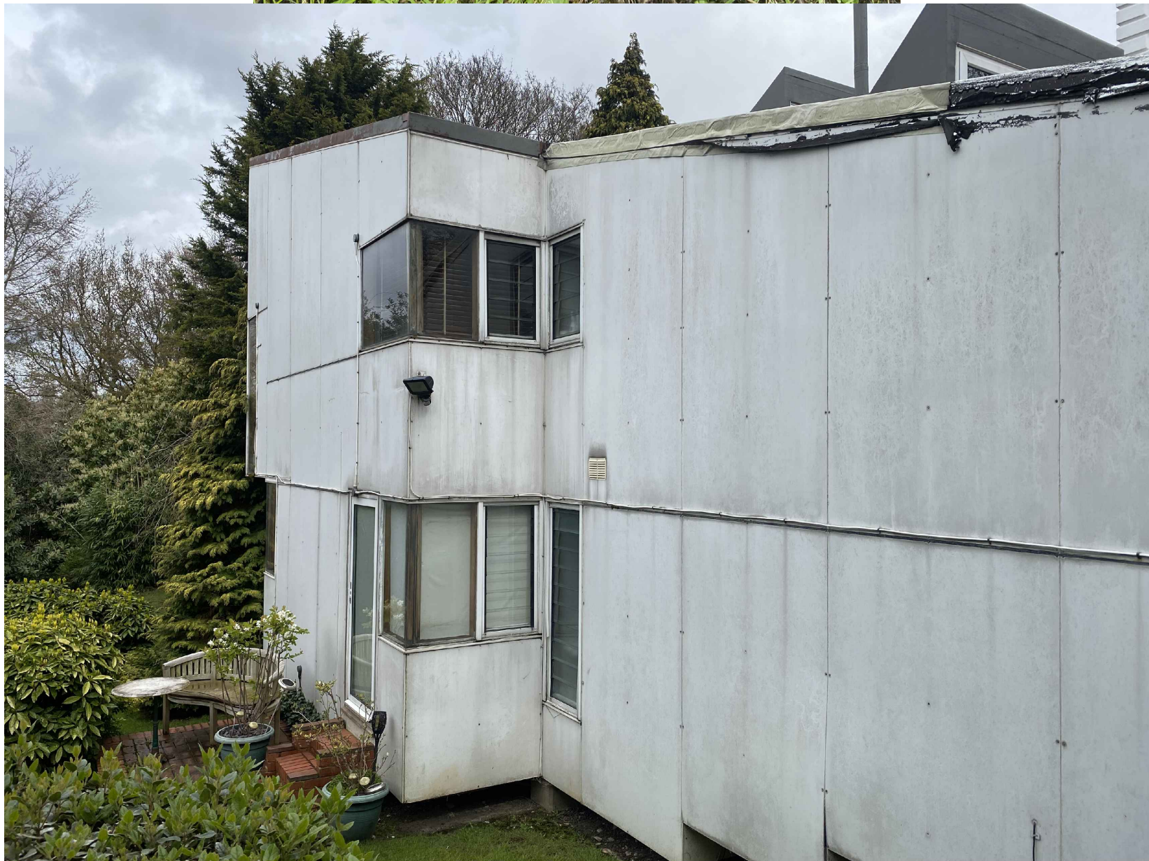
EXISTING DILAPIDATED WHITE CEMENT BOARD CLADDING
