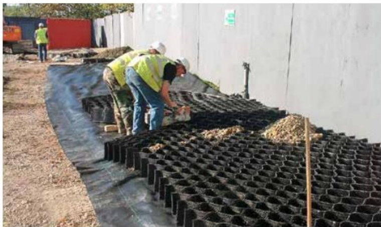
SGN 3-06 Cellular products are a very effective means of providing ground protection where heavy vehicle use is expected. Here, it is being used to temporarily widen an existing road, to be removed once the construction is finished.
