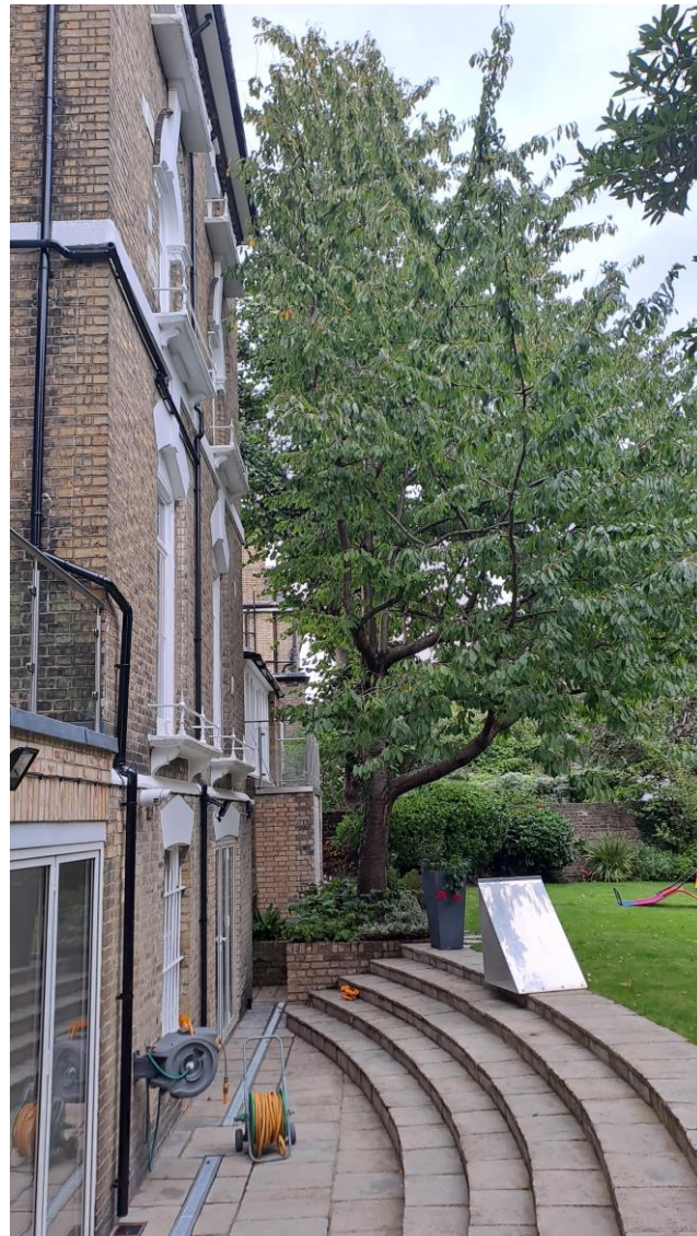
Photo 1 looking west at T1 cherry showing the curved steps and retaining wall.
