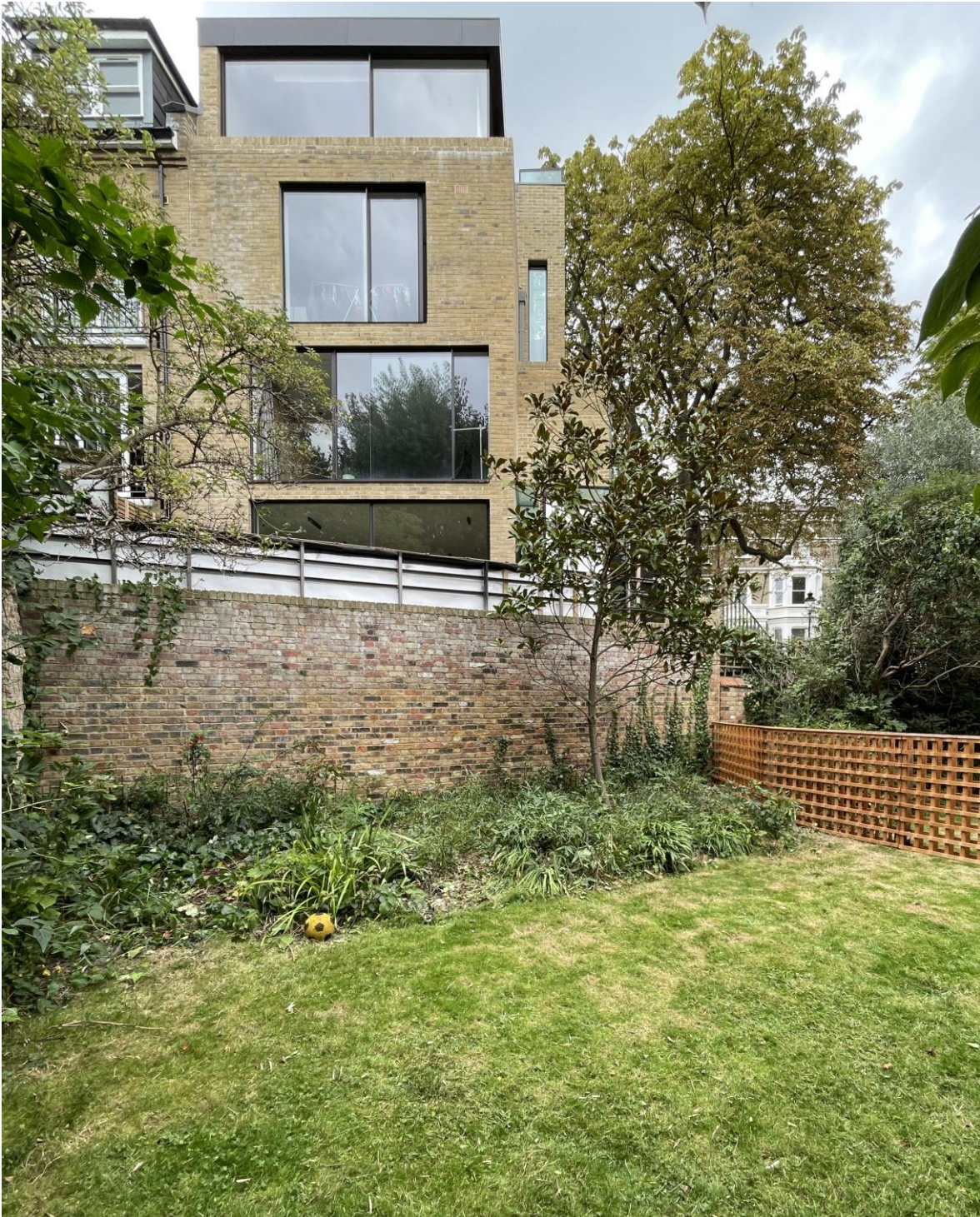
Existing Photo of the rear elevation
