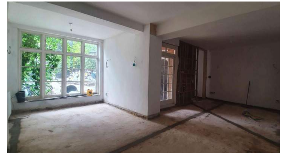
View B: Existing concrete slab, masonry wall (plastered) & stud wall in background
