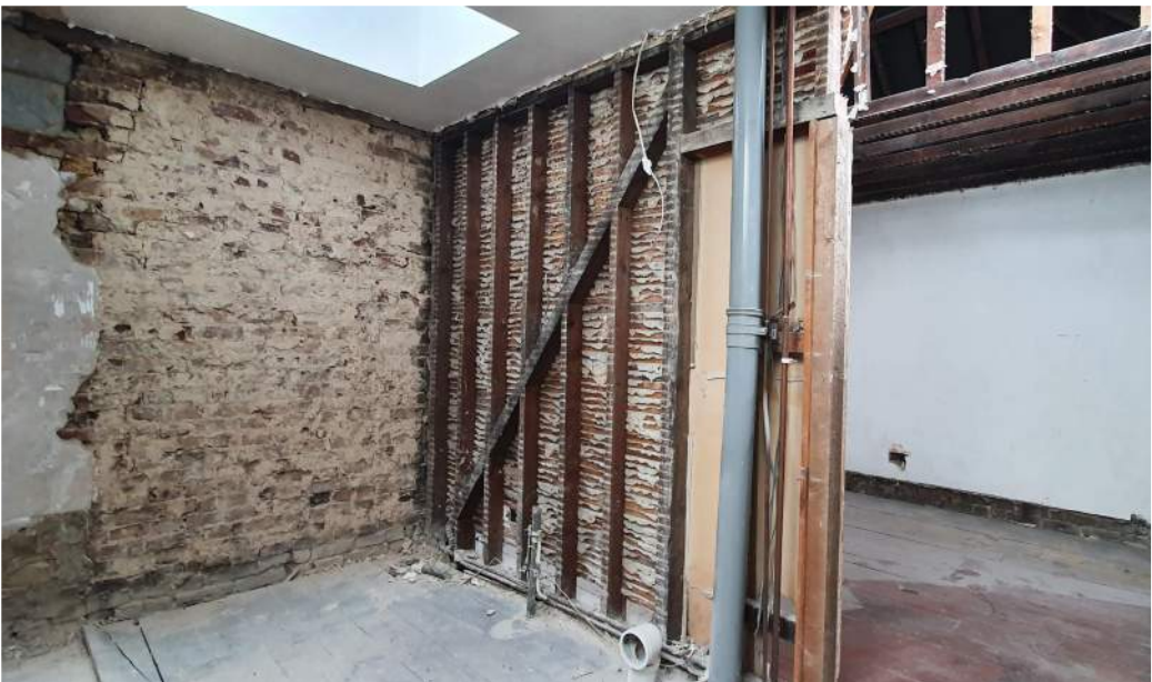
View A: Masonry walls & older stud wall
