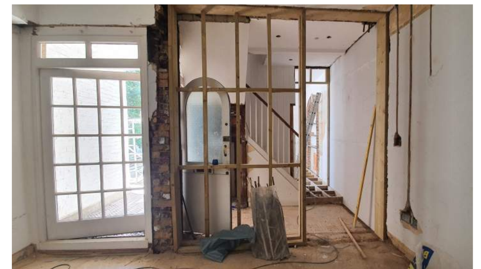
View C: Timber stud wall, masonry wall, raised floor in background
