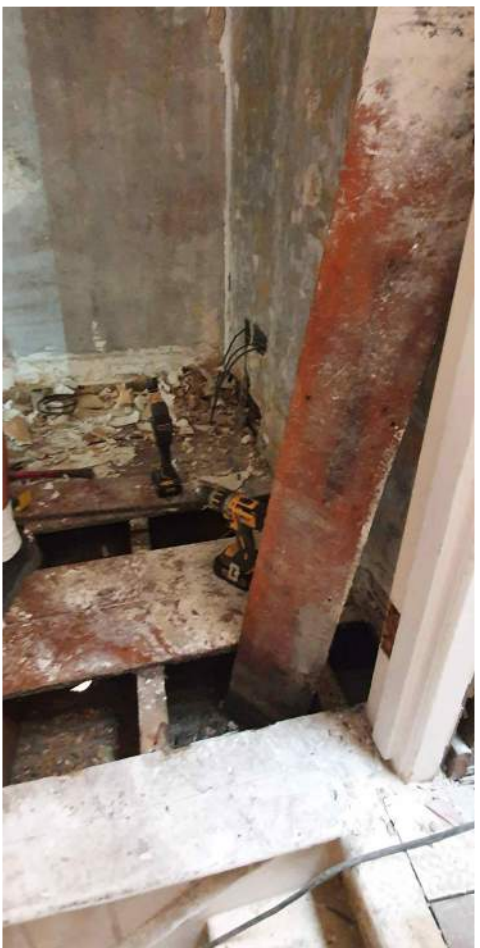
View C: Timber floor joists
