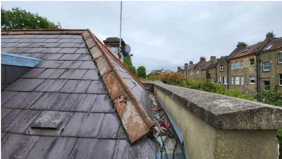
View A: External Roof showing slates, ventilation slates & coping stones
