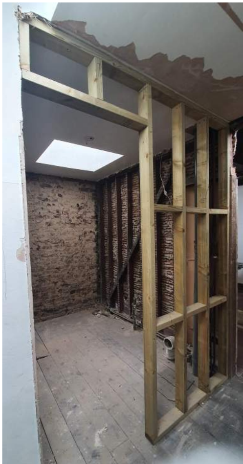
View B: Newer timber stud wall & floorboards
