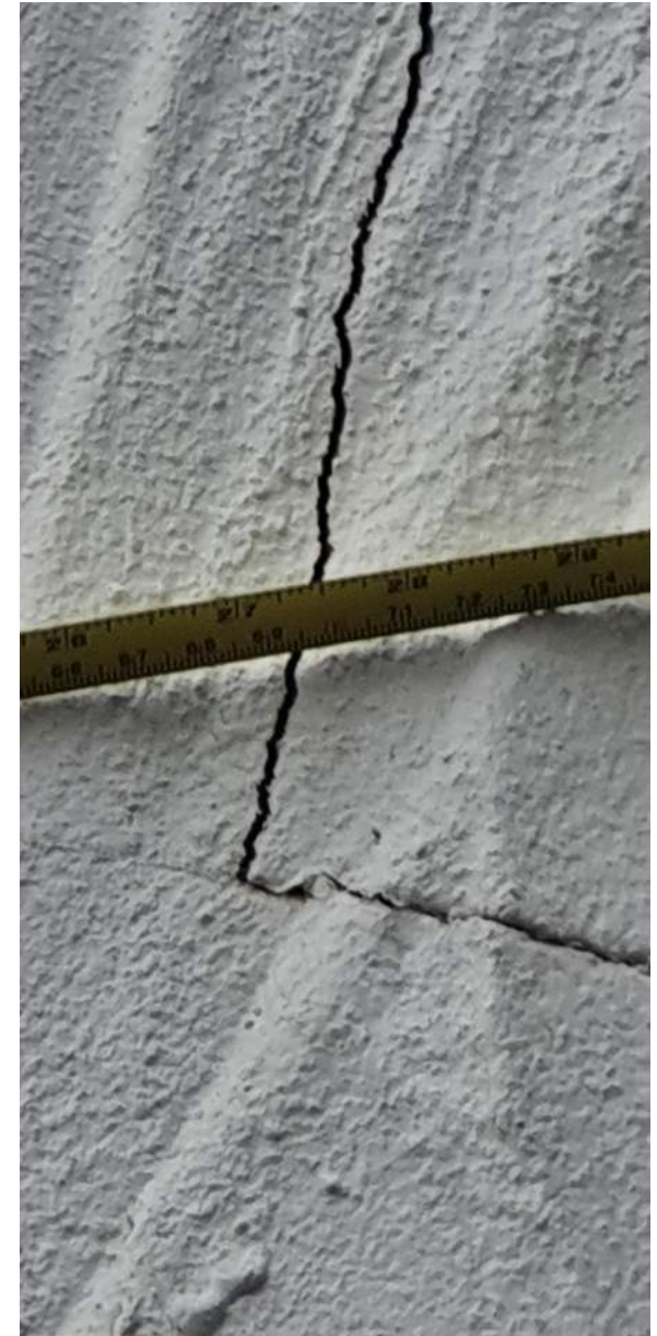
Figure 11:- East Elevation detail of crack
