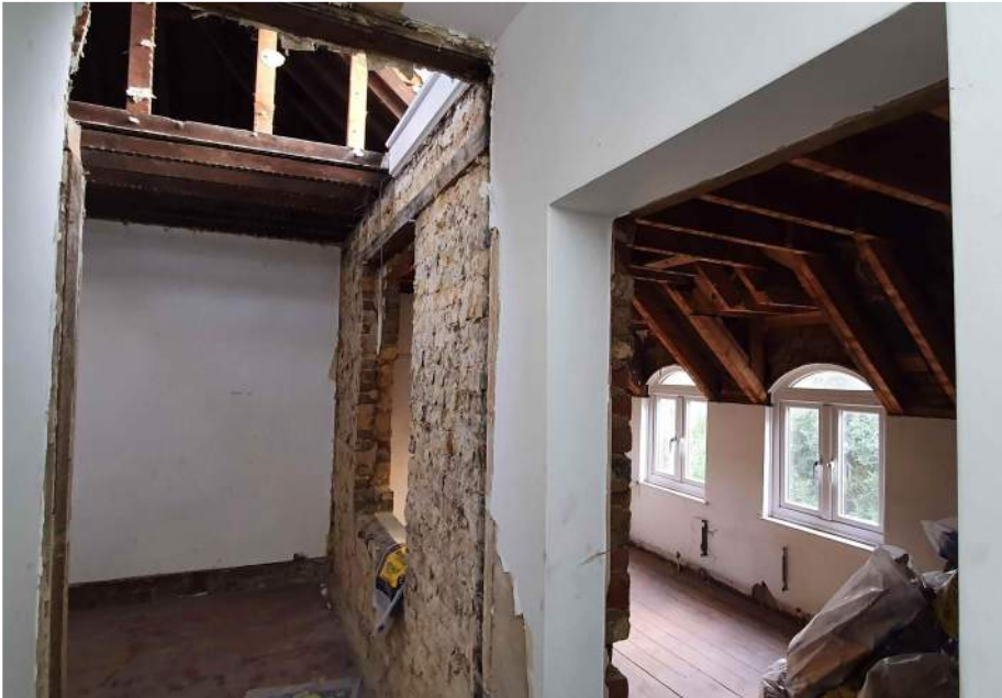
View C: Roof Type 2 (LHS), Ceiling Joists & Roof Type 3 (RHS) Note: Masonry partition wall and ceiling joists in photograph now removed
