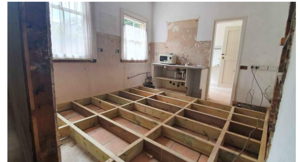
View A: Terracotta tiles, raised timber floor, masonry & stud wall (plastered)
