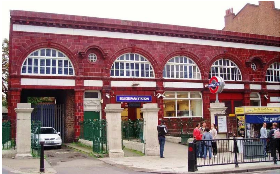
Belsize Park Station, 1907 Architect: Leslie Green
