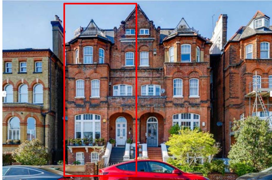
22 Belsize Lane, front facade
