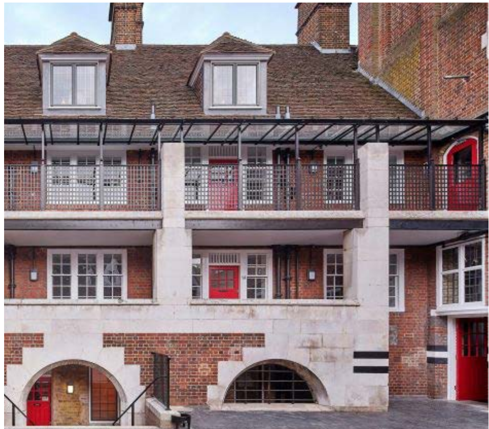
Belsize Fire Station, 1914 Architect: Charles Canning Winmill
