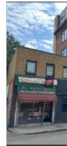
Photograph of Existing Shopfront
