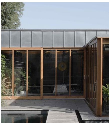
Zinc cladding and treated timber windows Garden Room by Hugh Strange Architects
