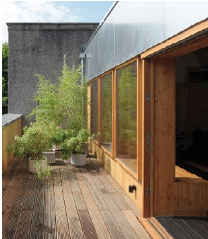
Treated timber windows and timber cladding. Clapton House by Hugh Strange Architects
