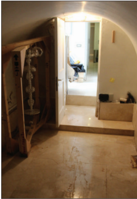
Plate 5. South vault, looking West.
