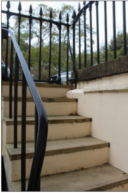
Plate 1. Exterior, steps, looking North-west.
