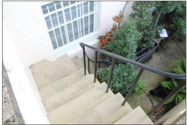
Plate 2. Exterior steps, looking South-west.
