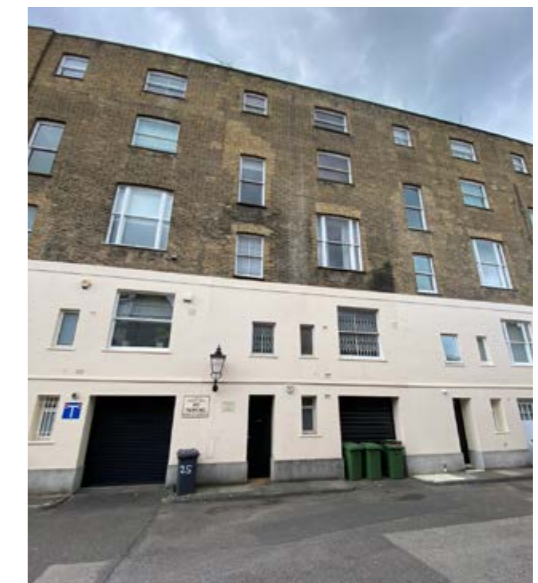
Lower Ground Rear of House
