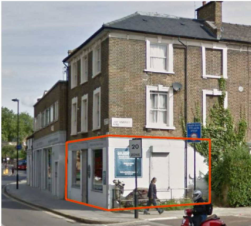
Fig.1 Street View of No. 74 Highgate Road, London - Site outlined in red
