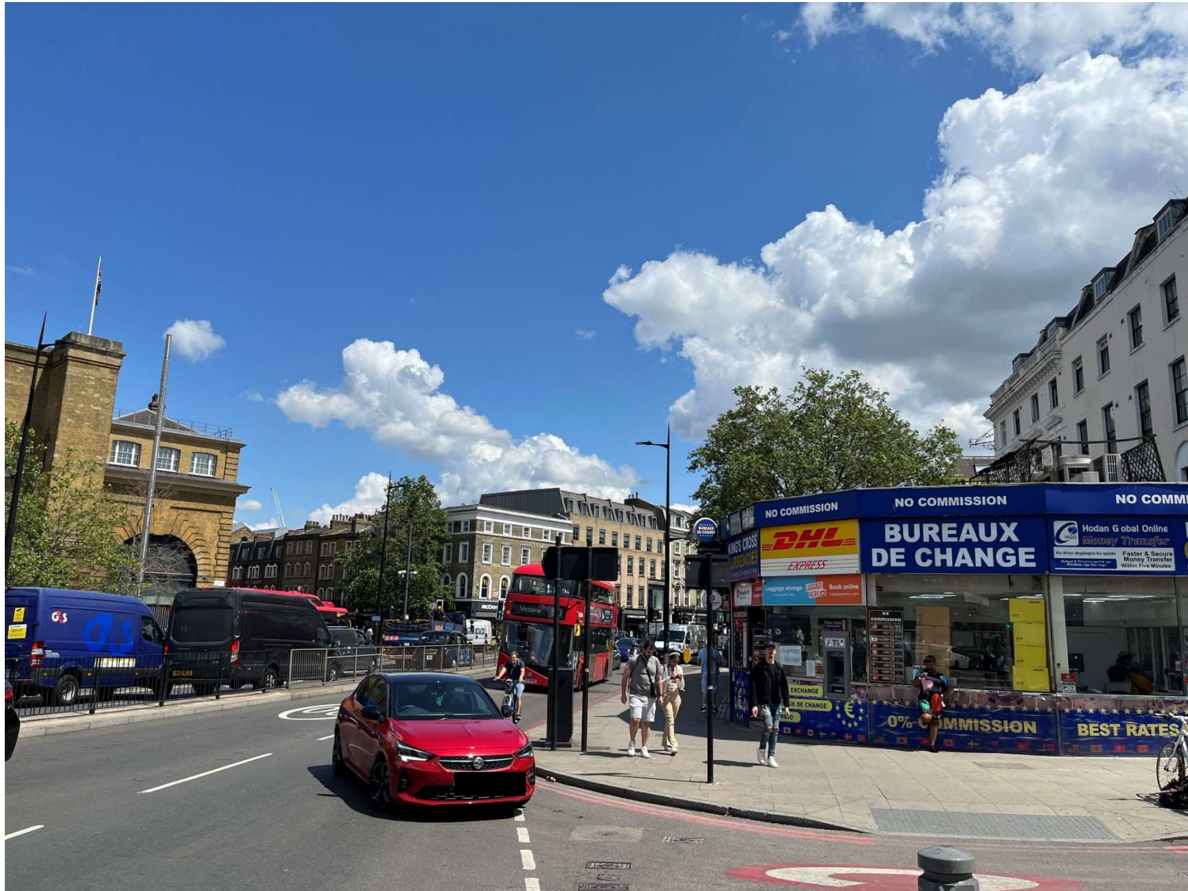
View East along Euston Road toward main junction (Kings Cross Station to left, frontage and hotel adjoining the proposal site is to the right)
