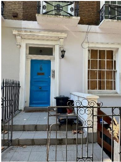
Fig.11 Arlington Road street view
