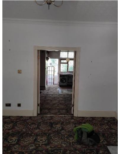
fig.16 view towards kitchen
