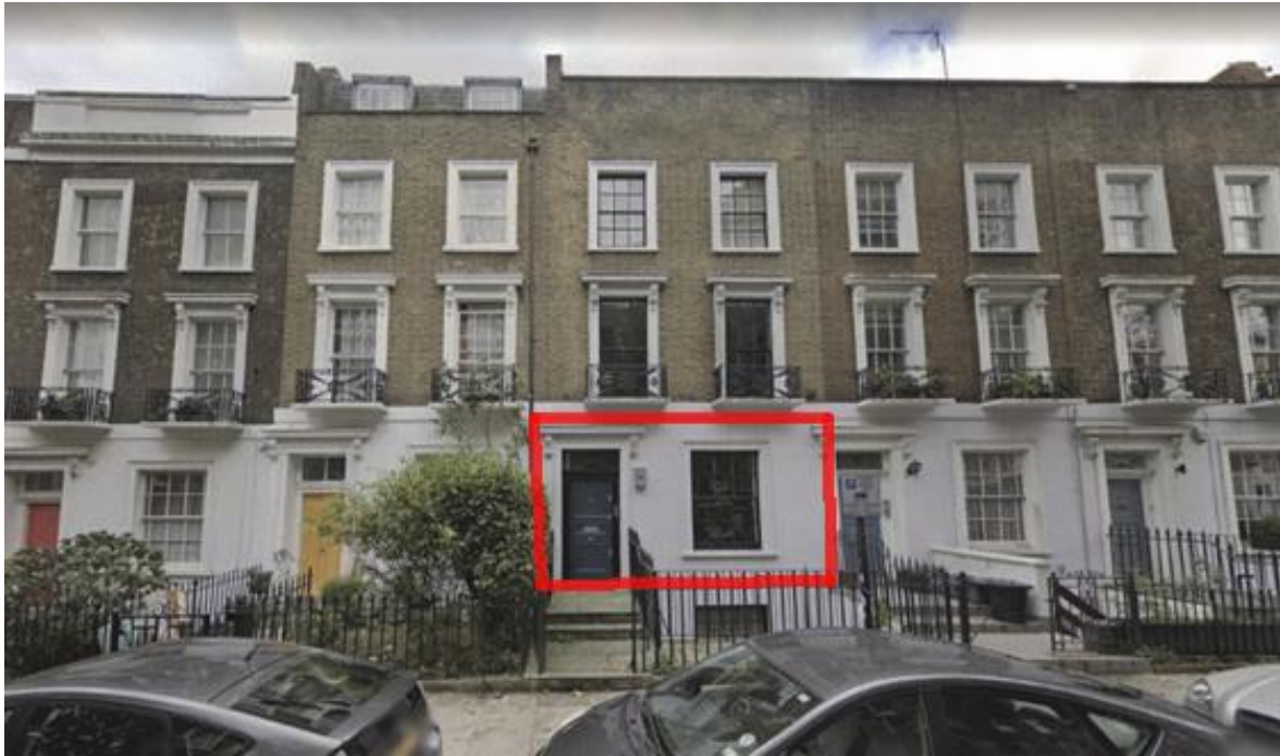
Fig.4 Street view of Arlington Road
