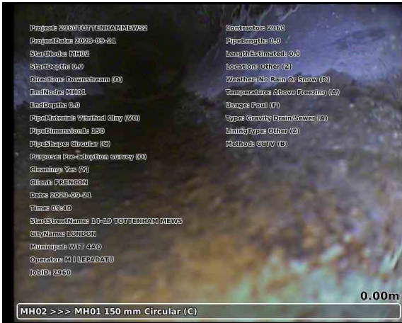
20230921-094051-snap0000.jpg, 00:00:00, 0.00 m Start node, manhole, reference: MH02
