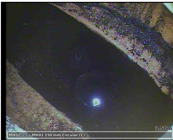
20230921-094051-snap0002.jpg, 00:00:20, 3.50 m Finish node, major connection without manhole, reference: MH01
