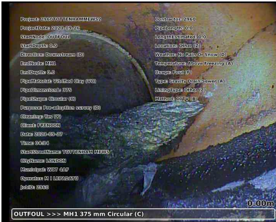
20230927-163711-snap0000.jpg, 00:00:02, 0.00 m Start node, outfall, reference: OUTFOUL
