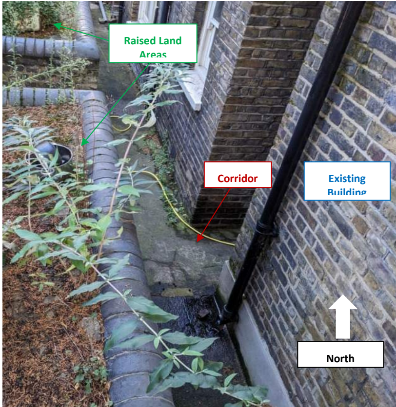
Plate 2. Rear of the existing building – corridor and raised land areas
