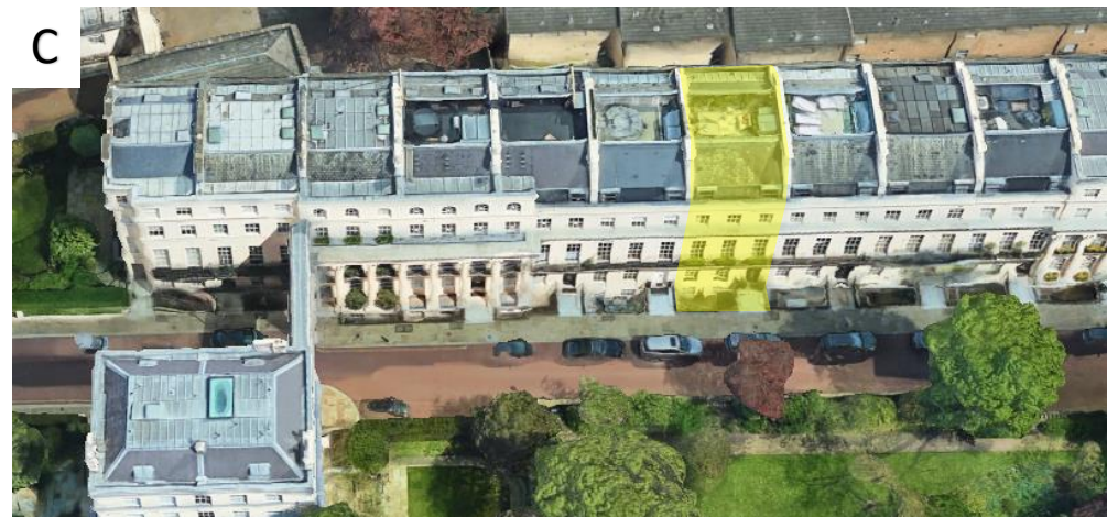
The view of Front of building – facing East – with No.34 highlighted..
