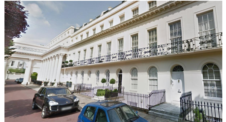
2.) View of similar works at No.26 – (currently under construction)
