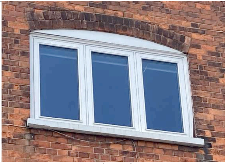
Window no. 3 - EXISTING
