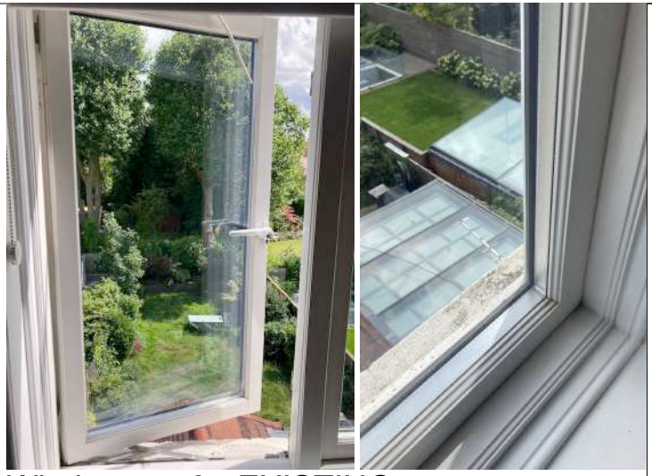
Window no. 3 - EXISTING
