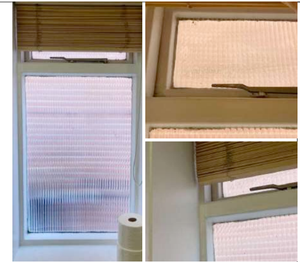
Window no. 2 - EXISTING
