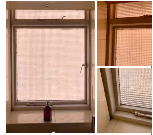
Window no. 1 - EXISTING
