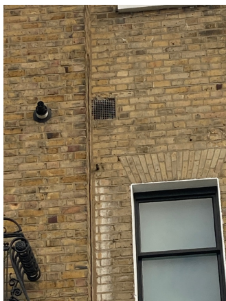
6. Plastic grille on front elevation at 44 Fortress Road
