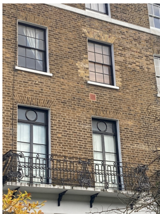
7. Airbrick on front elevation at 48 Fortress Road
