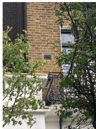
8. Cast iron grille on front elevation at 52 Fortress Road
