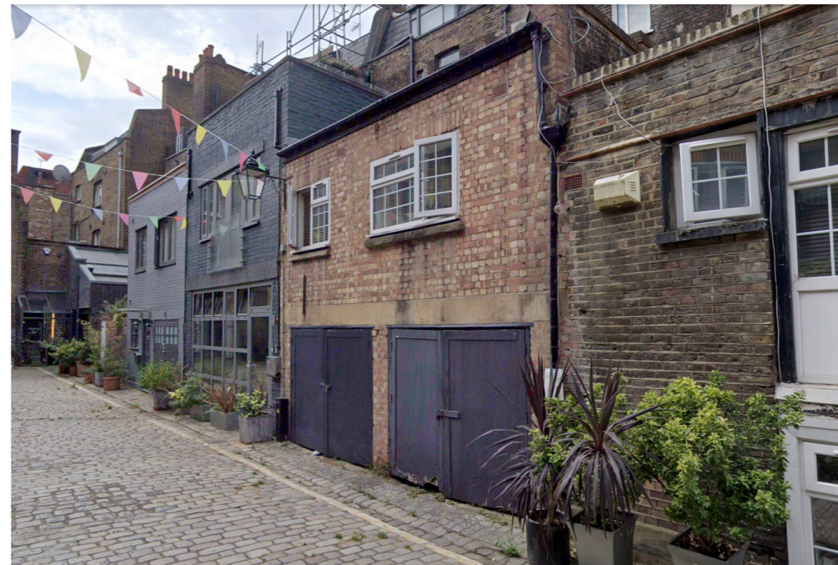
View South showing properties along the West side
