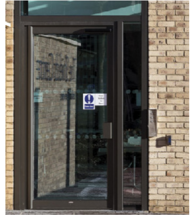
AA720 thermally broken aluminium manual swing doors
