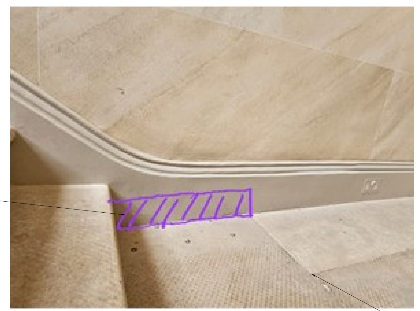
PHOTO P1 VIEW OF SKIRTING BOARD AT LANDING LEVEL.
