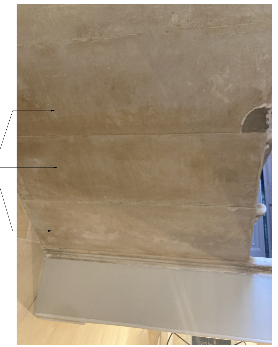
PHOTO P2 UNDERSIDE VIEW OF STAIRS
